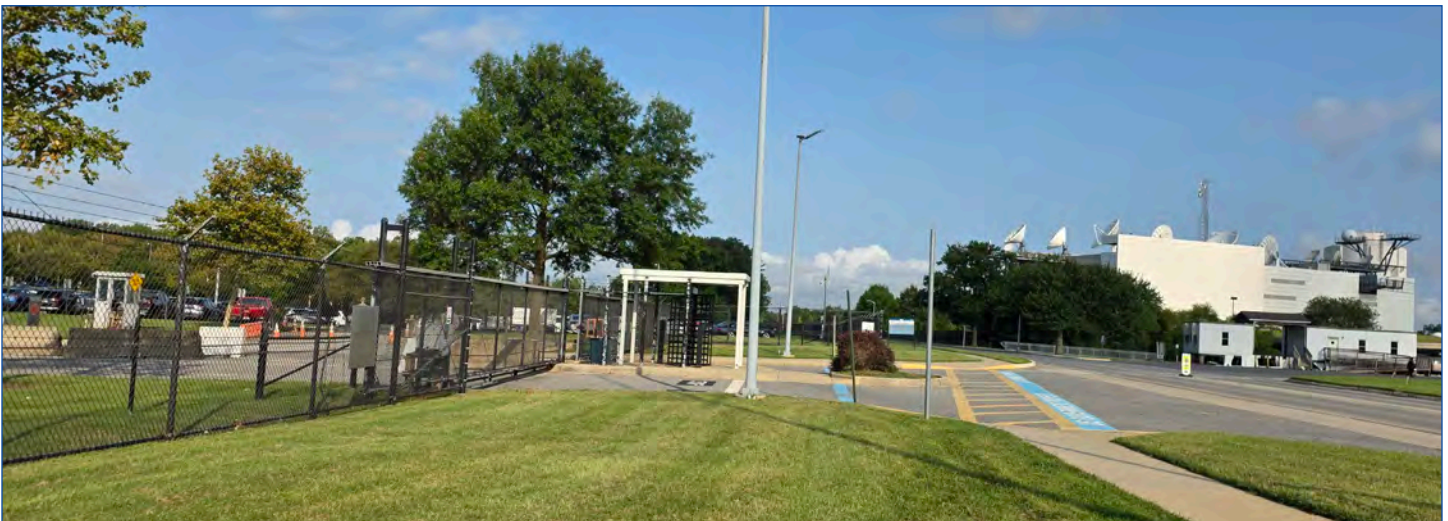
NSF Suitland Staff Access Gate
