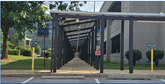
Covered Path to SFC Gate 7 from Suitland Metro Station Source: Marstel-Day/The Diallo Group Planning Team
