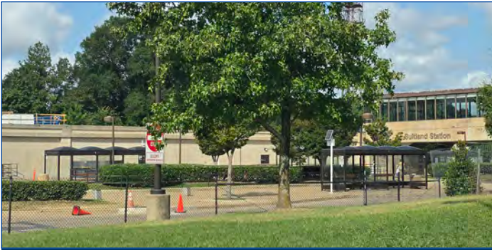
Bus Bays at the Suitland Metro Station Source: Marstel-Day/The Diallo Group Planning Team
