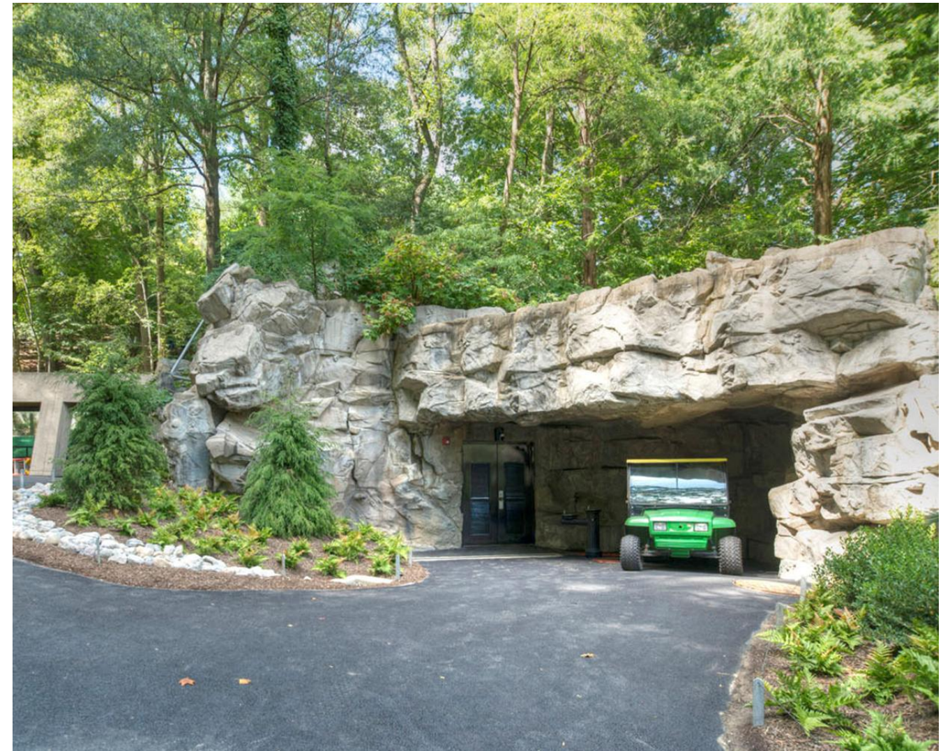
LSS building with volunteer trees growing on existing green roof
