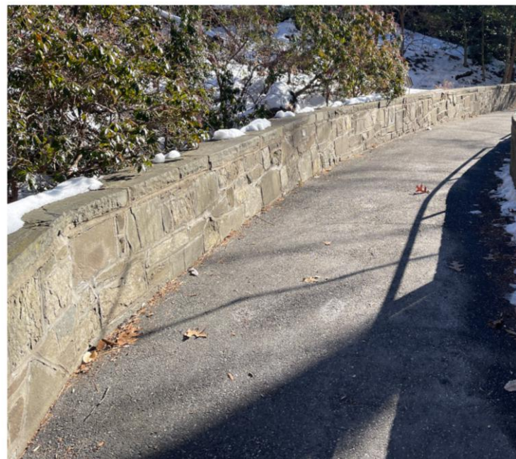
REFERENCE IMAGE FOR PROPOSED SITE WALL: Existing stone clad retaining wall
