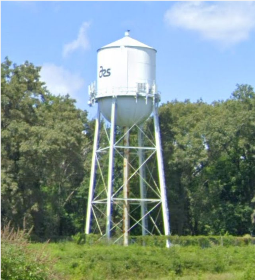
Enlargement of existing water tower
