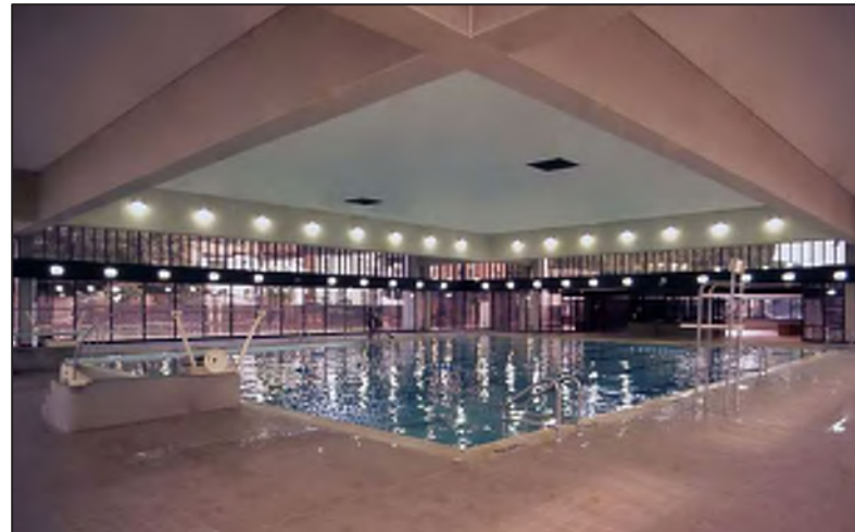
Figure 5: Interior of Capitol East Natatorium following completion (Delmar Architects)
