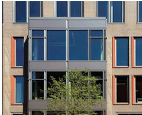
360 7th Street Southeast DC
