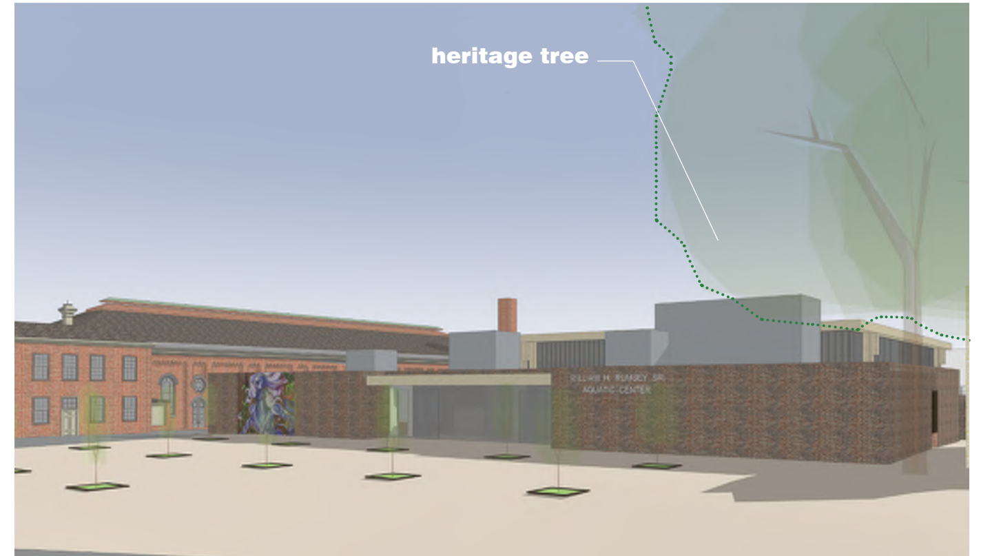
EXISTING VIEW TOWARDS EASTERN MARKET
