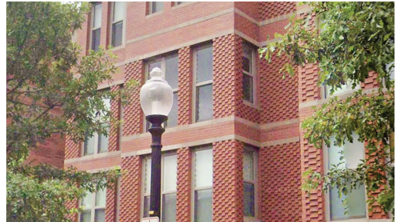
Brick Pattern btwn windows and contrasting brick bands
