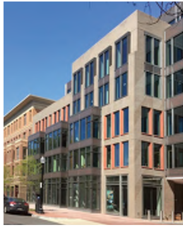
7th Street Southeast DC
