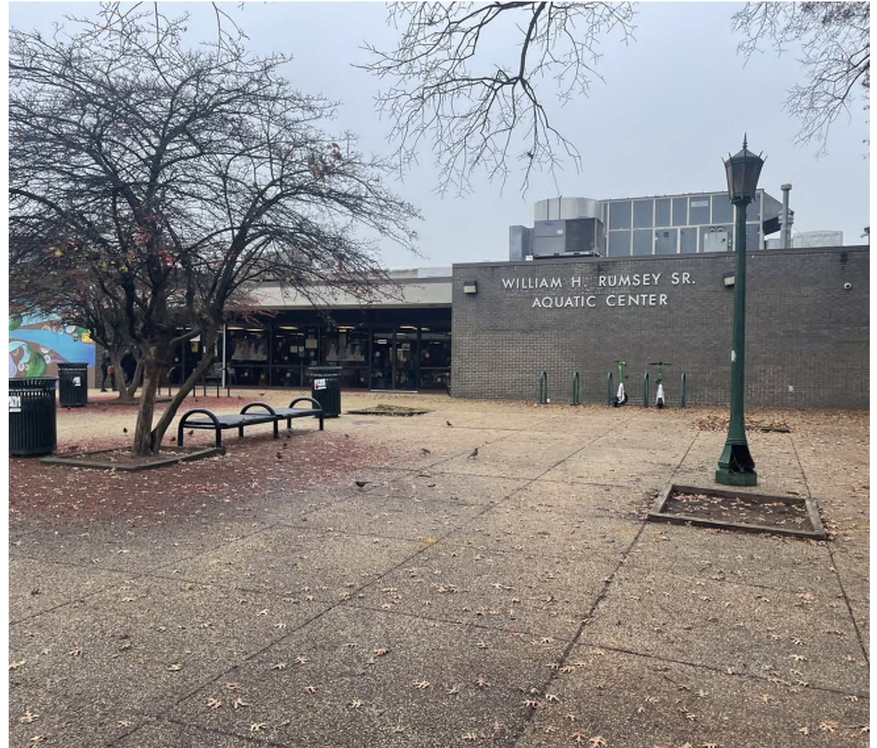
EXISTING AQUATIC CENTER ( TO BE DEMO'ED)
