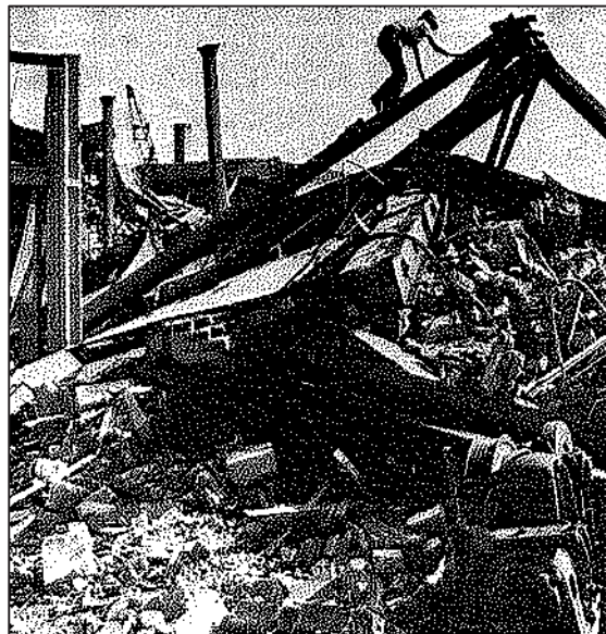
Figure 2: Demolition of Firehouse No. 8 in preparation for construction of Capitol East Natatorium (The Washington Post)
