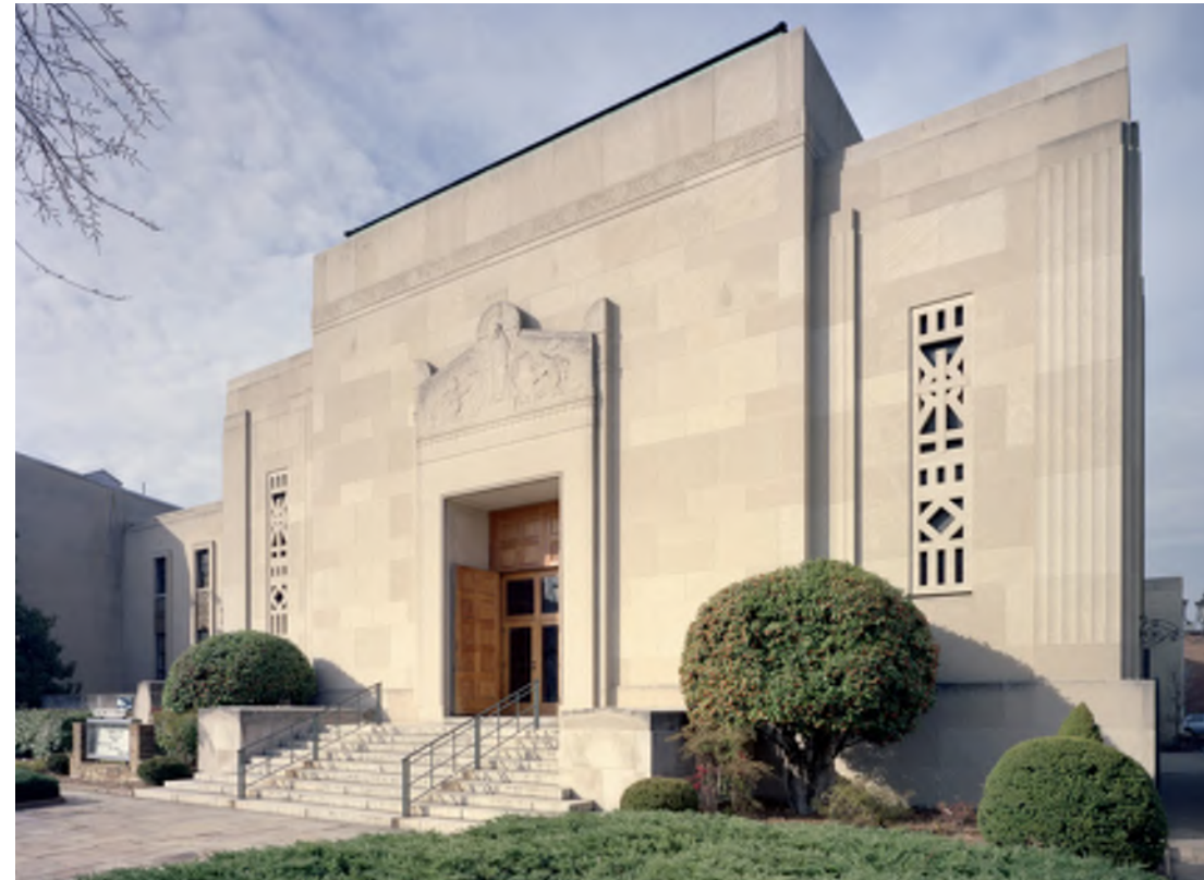
Grand entry vol, dbl-height windows, Restoration Church, Capitol Hill
