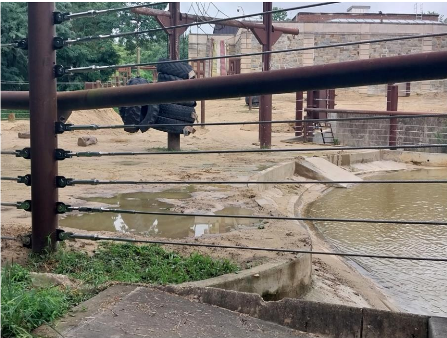
Photo of Yard 1 displaying ponding and runoff after a rain event.
