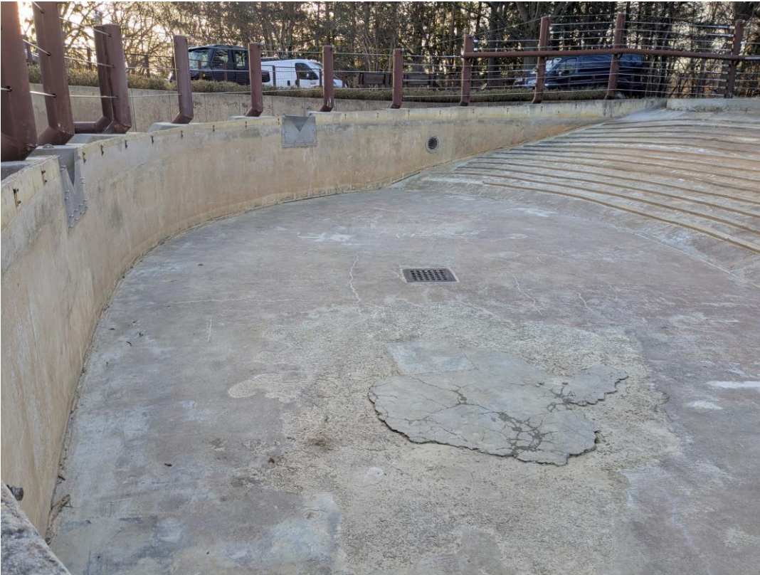
Photo of existing Pool 1 exhibiting concrete spalling.
