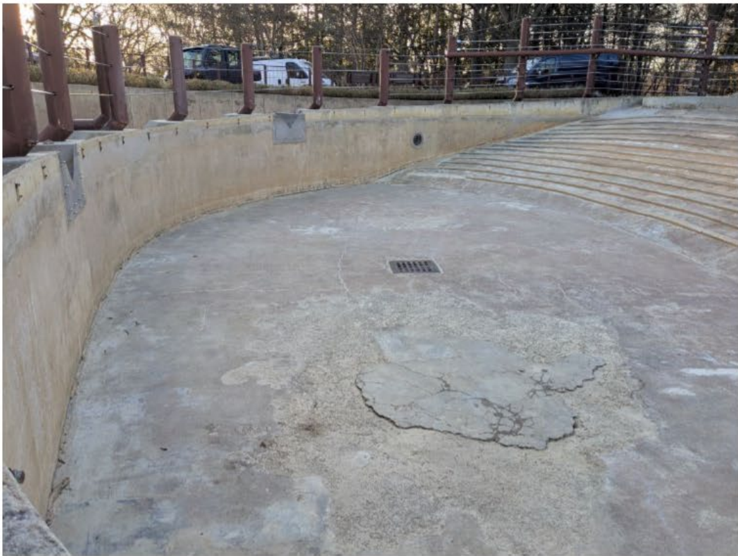
Photo of existing Pool 1 exhibiting concrete spalling.
