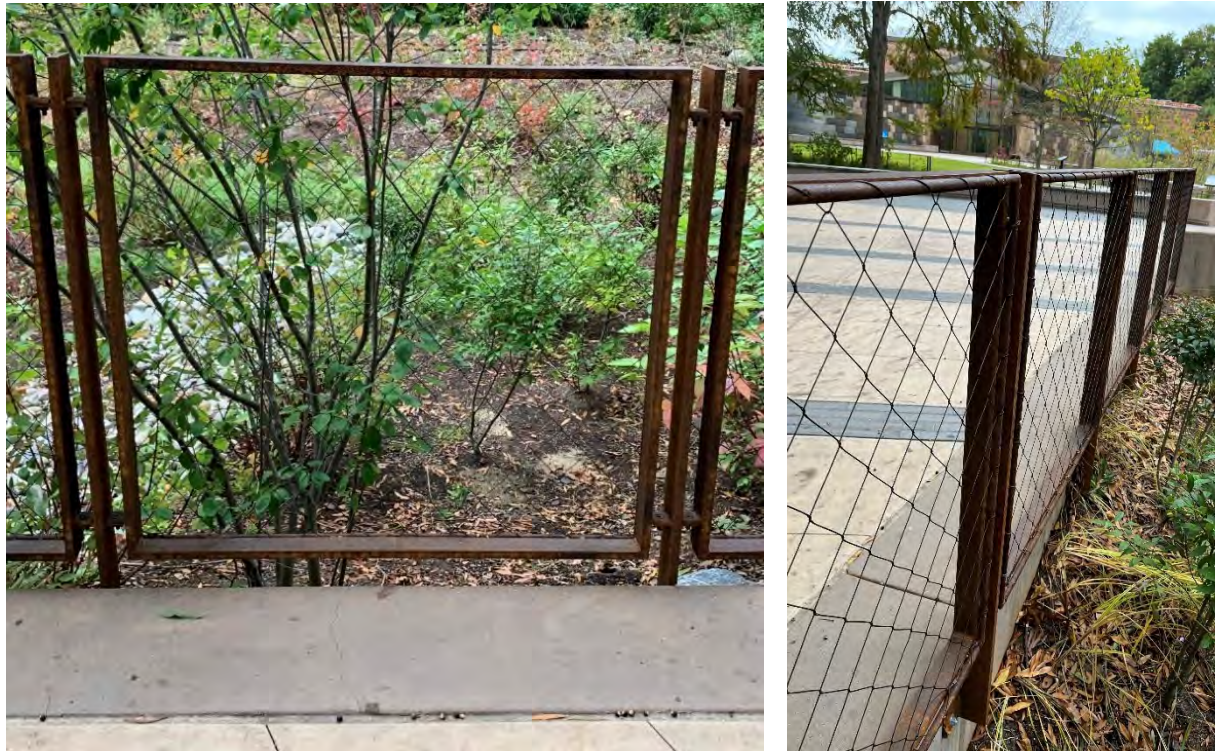
Example of face mounted weathering steel guardrail on Bird Plateau
