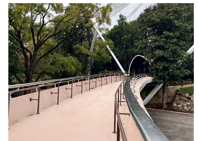
2017 Resurfacing and handrail addition to Great flight Aviary Bridge
