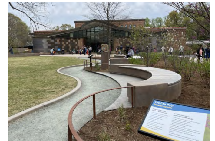
Crushed Stone walk at Bird House entry plaza
