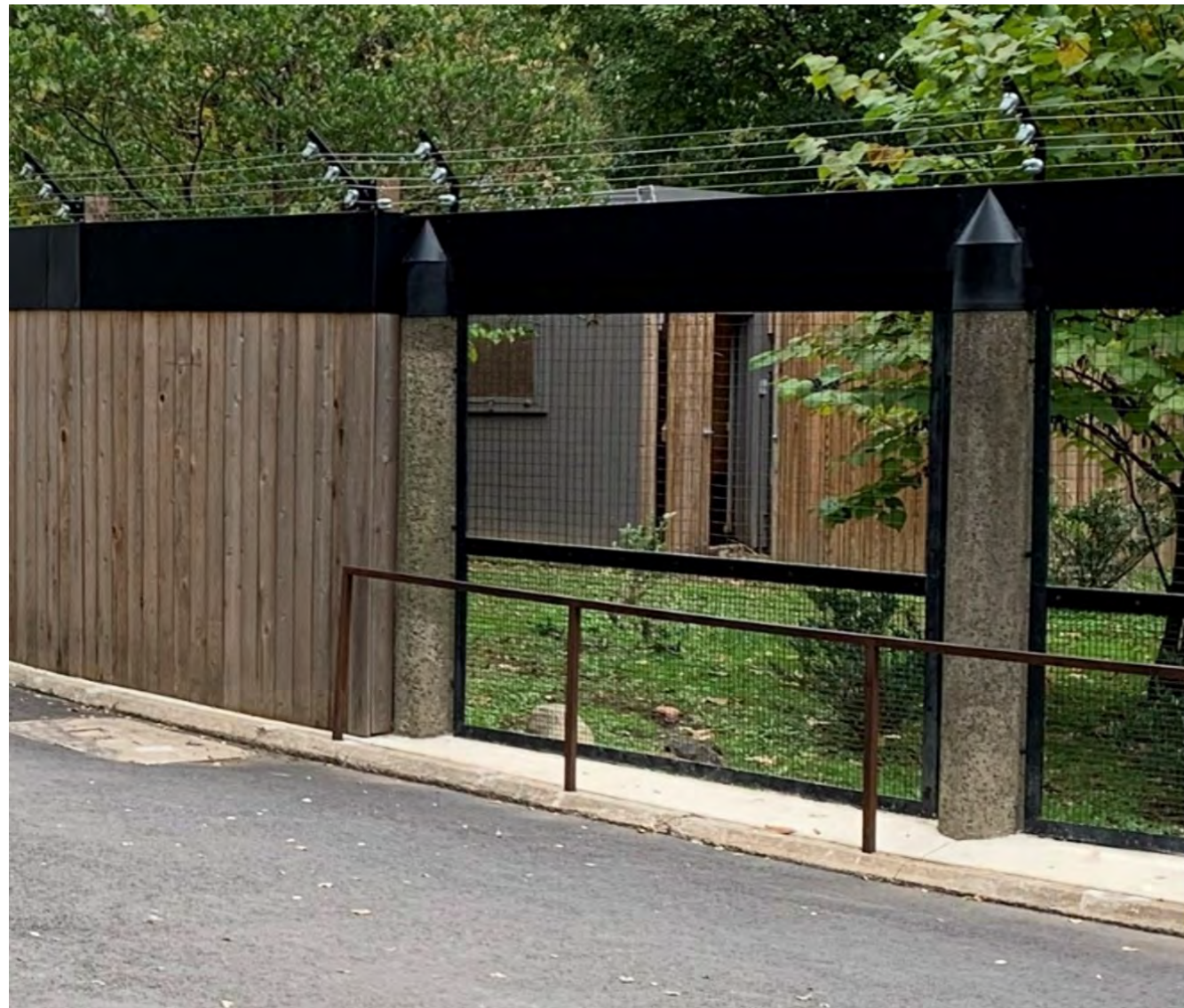
Exhibit fencing to match language currently installed at Bird Plateau Southern Exhibit Trail with added predator proofing.
