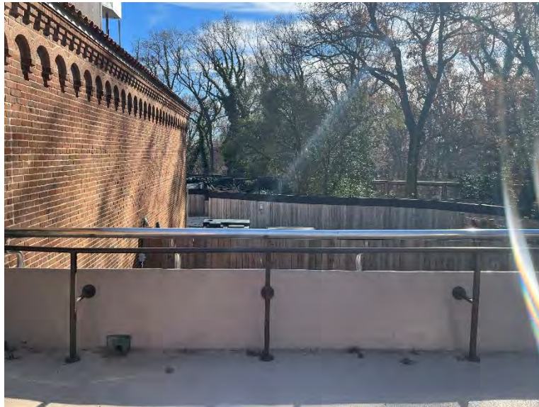
View from GFA Bridge looking at intersection location with new walkway
