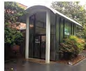
Entrance Vestibule, 1965 (photo 2013)
