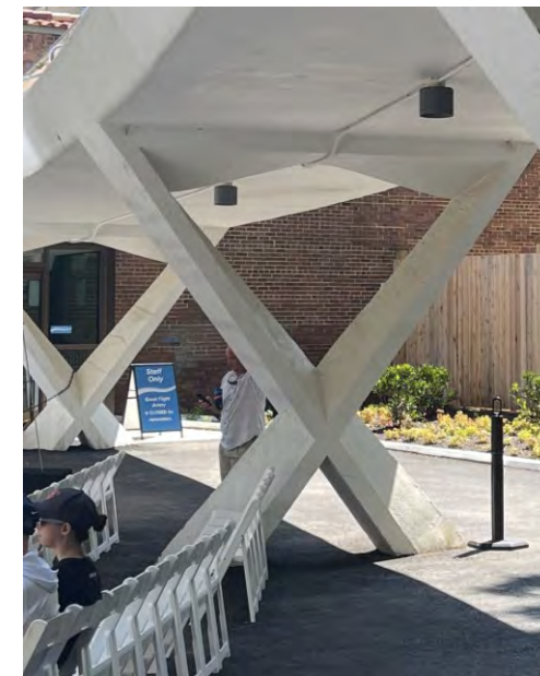
GFA Bridge upturned beam (Above). GFA Bridge supports (Below).
