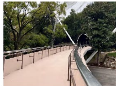
2017 Resurfacing and handrail addition to Great flight Aviary Bridge
