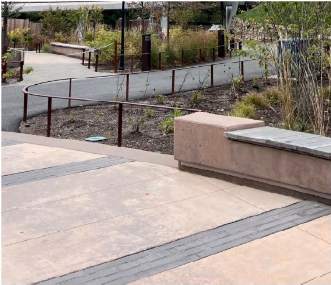
Dark grey linear pavers, stained concrete paving and bench, and kickrails to match language found in north plaza of Bird House
