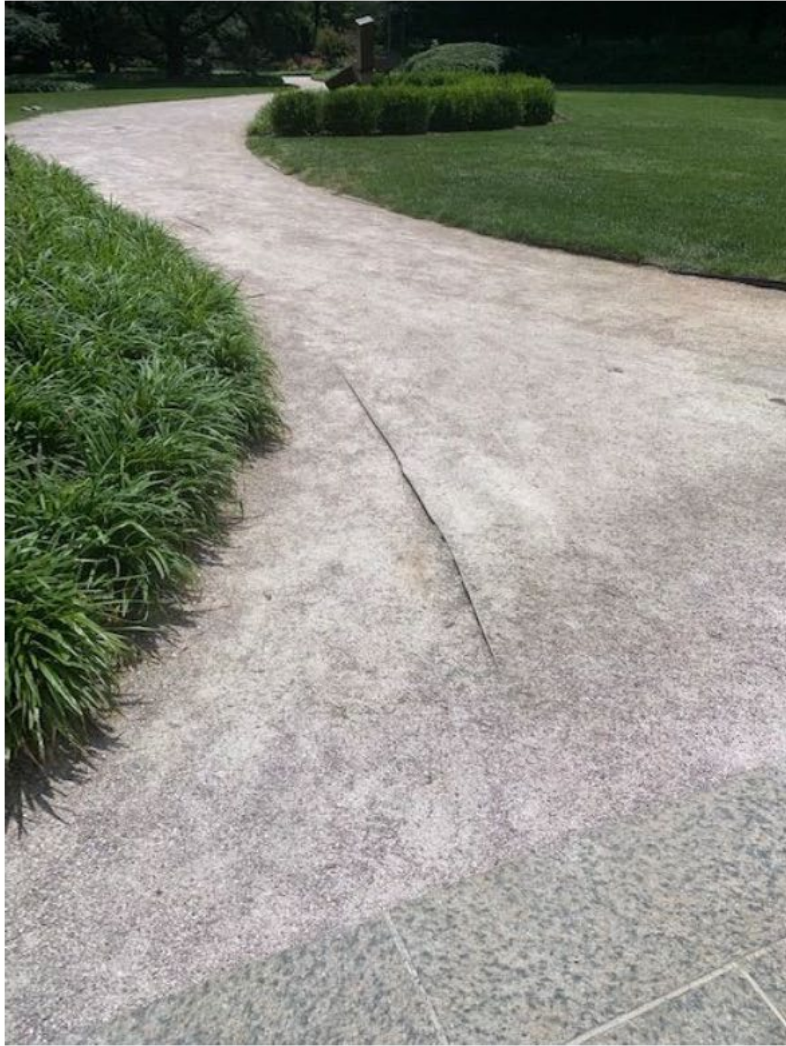
3. Gravel migration at gravel-path/ stone path intersection
