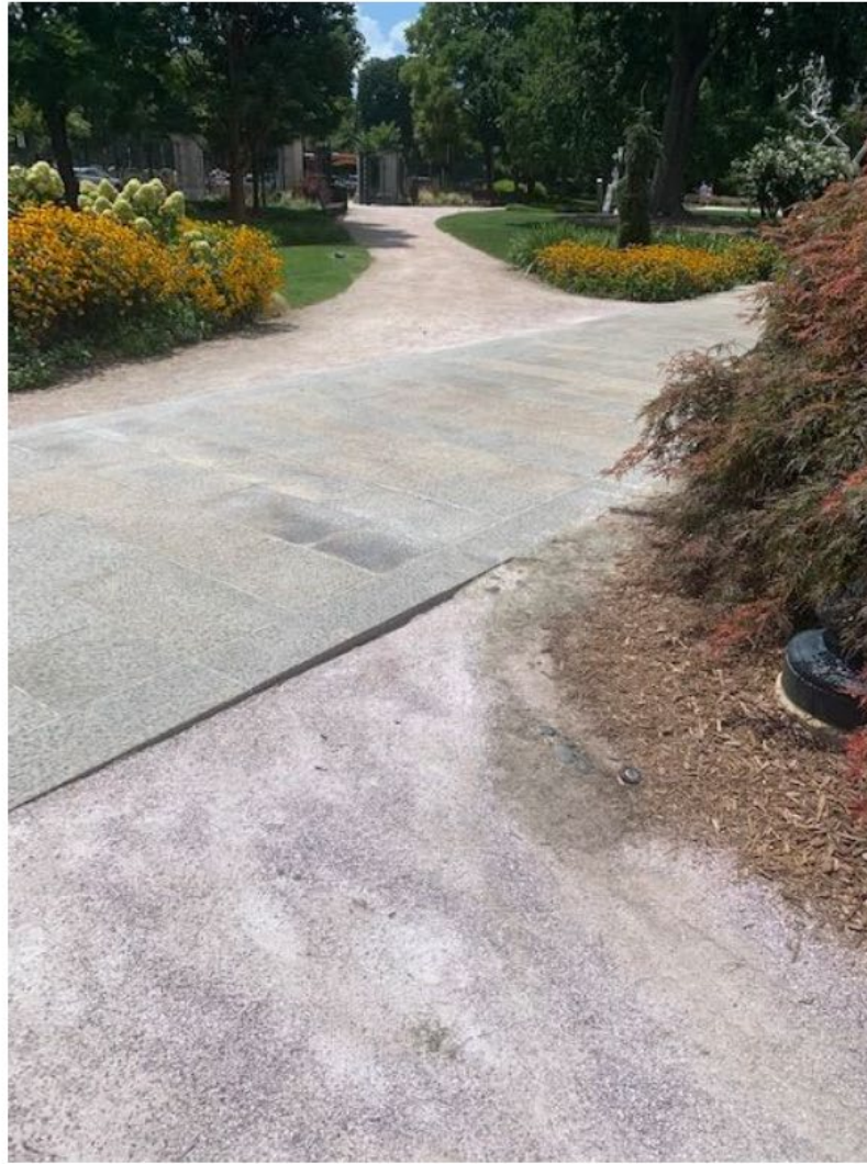
6. Gravel erosion at gravel-path/stone-path intersection
