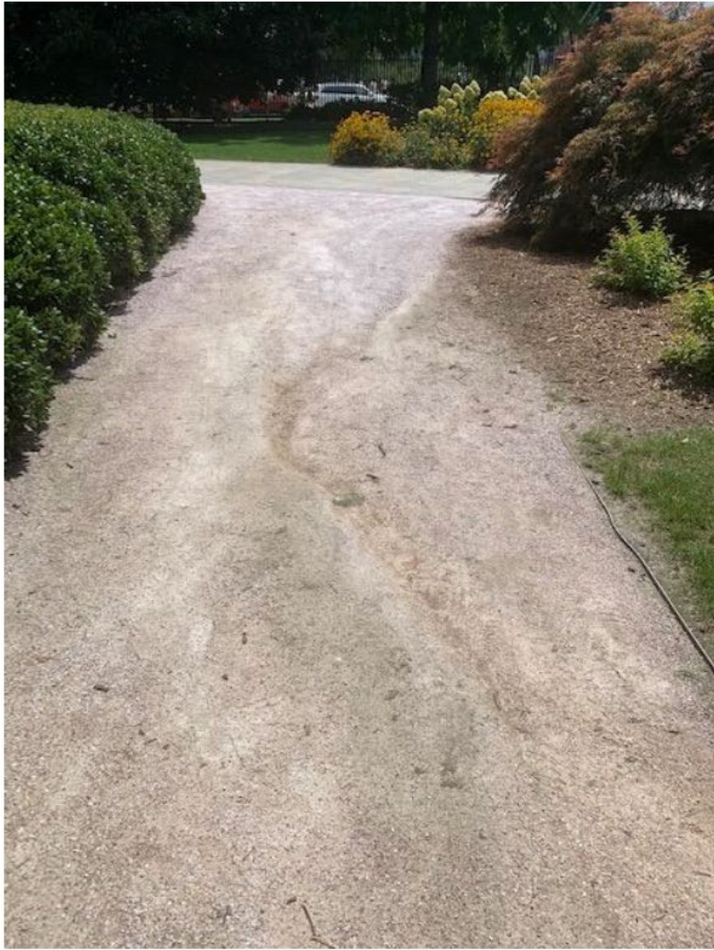
5. Gravel erosion along path
