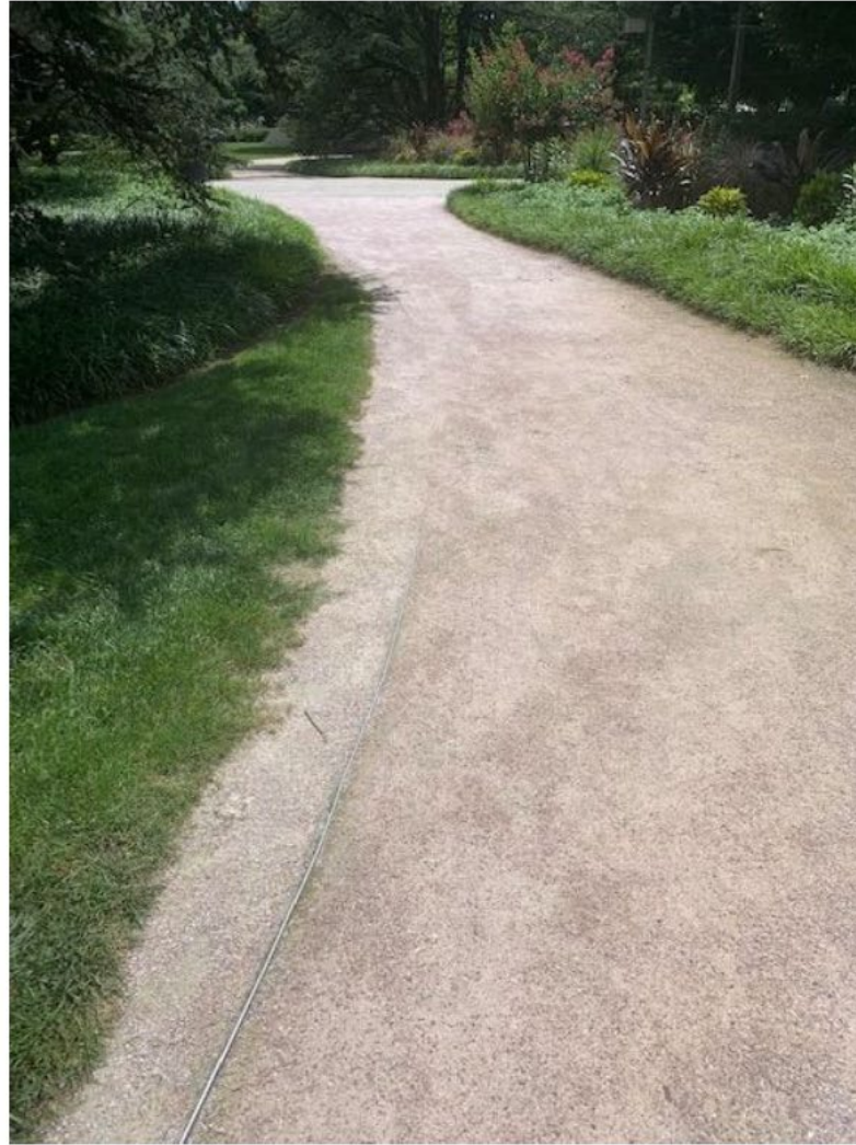
4. Gravel migration along gravel-path/ stone path intersection
