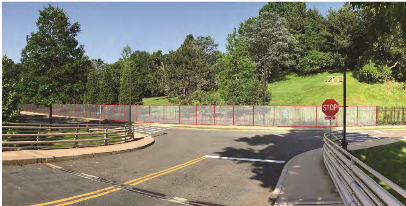
Proposed Location of Existing Ornamental Fence to be Replaced with Vehicle-Rated Fencing
