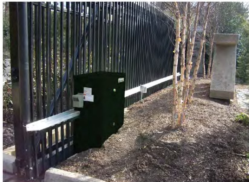
Figure 8c - Existing Ornamental Sliding Gate
