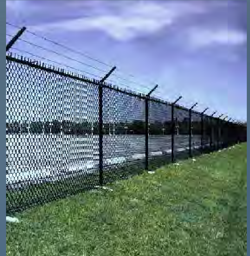
Example black plastic-coated chain link fence with three strands of black barbed wire
