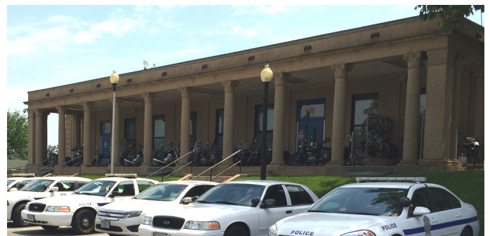
1.4 Existing USPP D-1 Station
