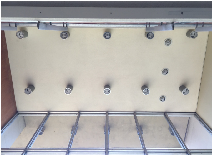
1.13 Character-defining light fixtures will be refurbished where possible or will be replaced in kind
