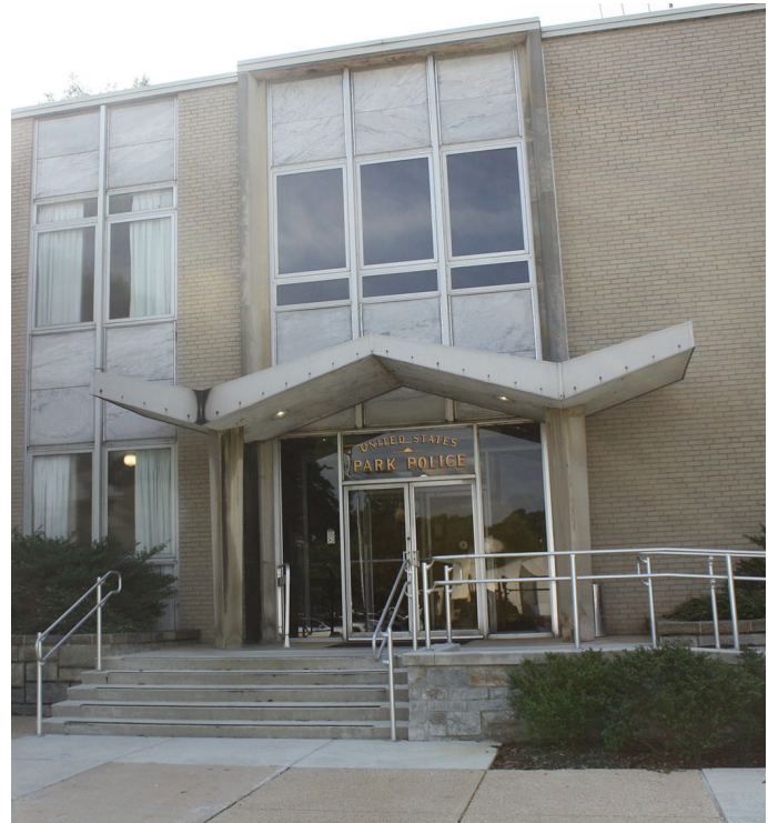
1.14 Entrance to Wing D, character-defining features will remain
