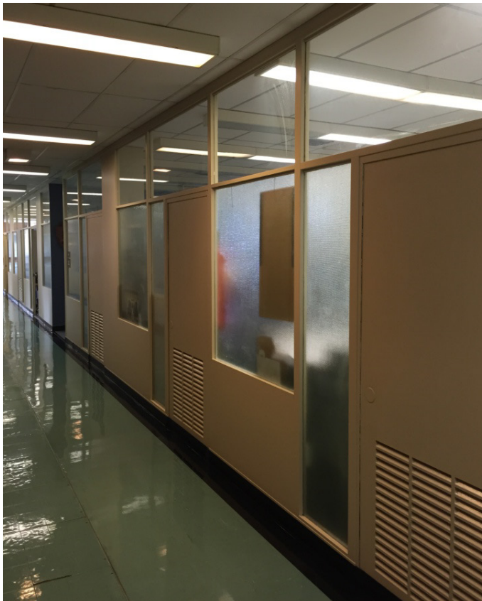
1.11 Existing partitions will be removed
