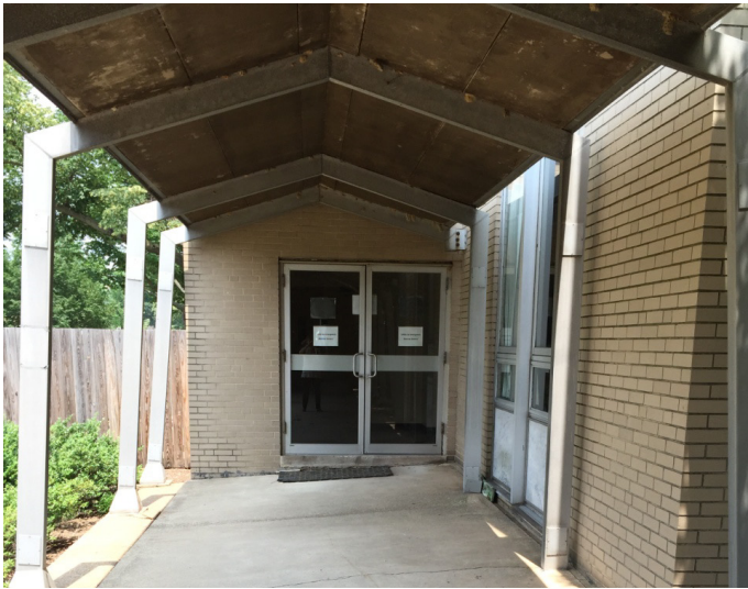
1.20 Existing condition of breezeway entrance to Wing A
