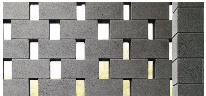
1.41 Masonry screen detail precedent
