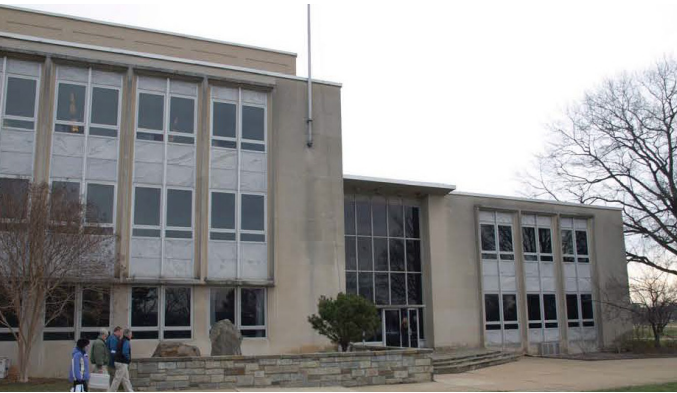
1.2 (Top) Existing USPP Headquarters, (Bottom) NCRO Wing A/B joined by atrium lobby.
