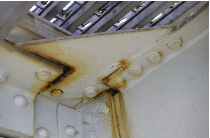
Image 3-62 Non-Welded Bracket, With Only Two Bolts Connecting The Tie Plate
