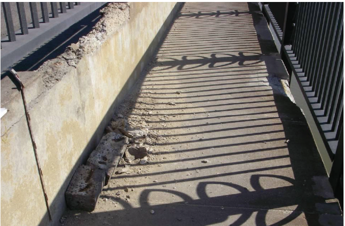
Image 3-59 Sidewalk Spall With Exposed Reinforcing Steel
