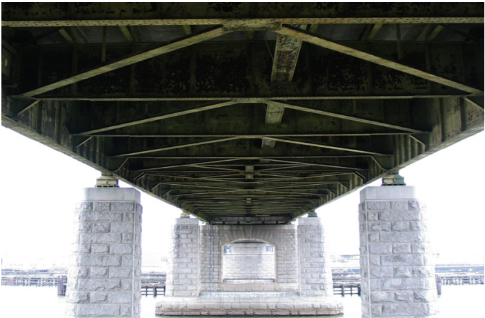
Image 3-58 Steel Corrosion On The Existing Frederick Douglass Memorial Bridge
