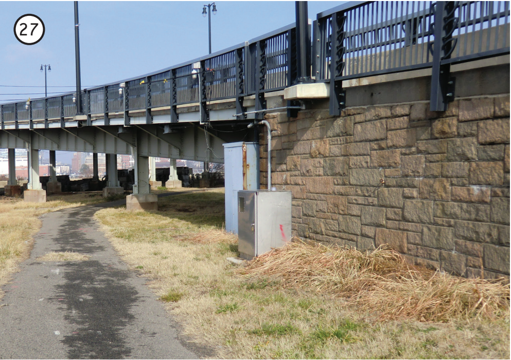
Image 3-28 Ashlar pattern stone retaining wall on South Capital Street
