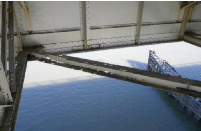
Image 3-60 Typical Swing Span Bottom Lateral Brace With Severe Deterioration
