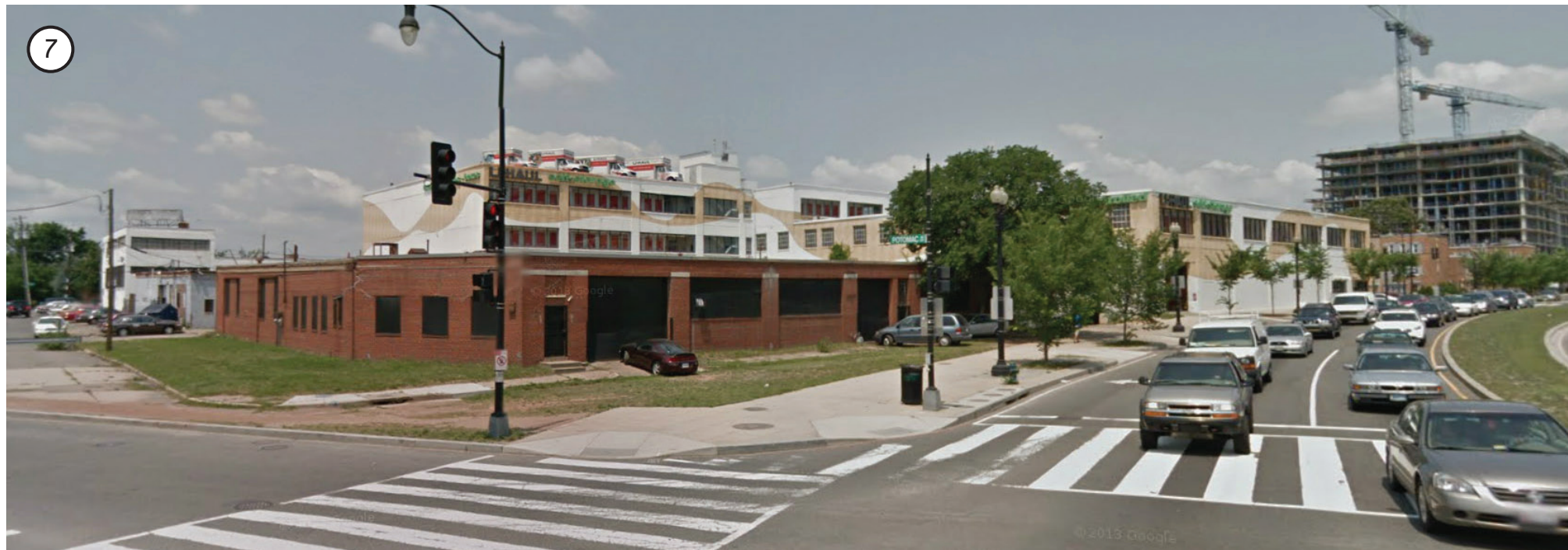
Image 3-8 Existing garage and UHAUL building
