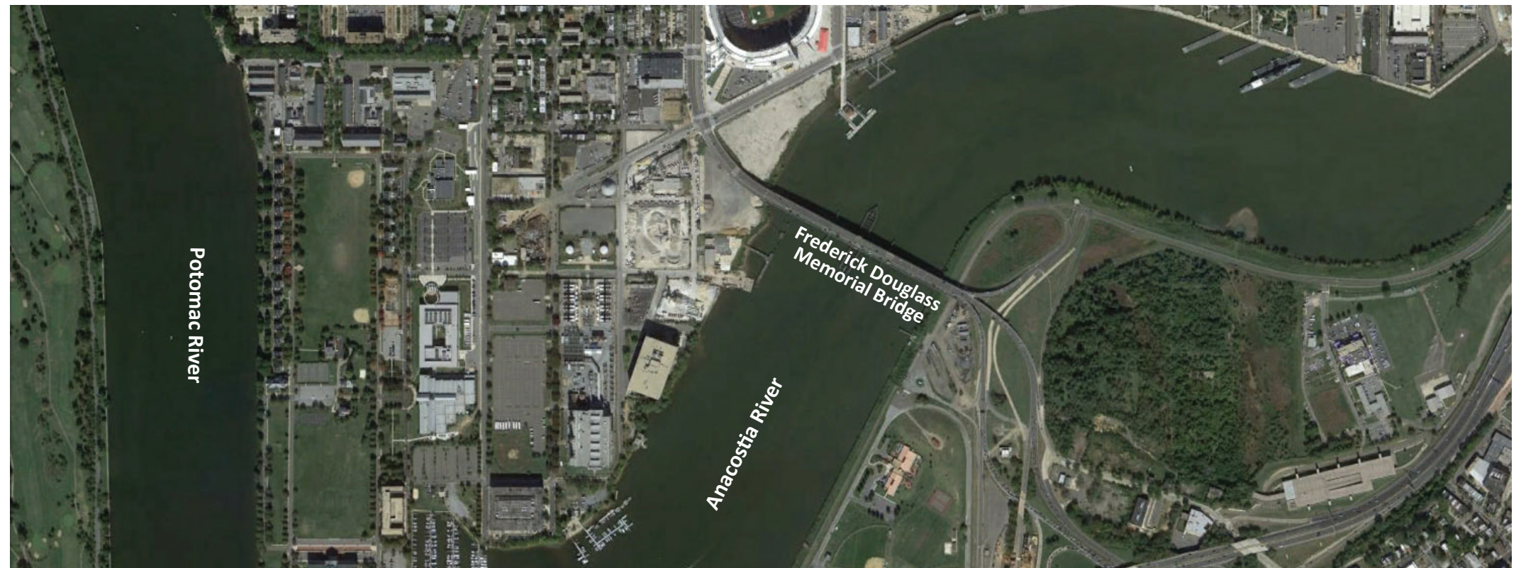
Image 2-2 Existing Frederick Douglass Memorial Bridge
