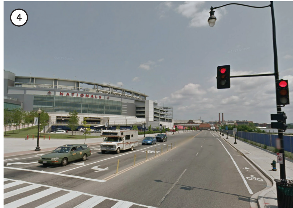
Image 3-5 South Capitol Street - Potomac Avenue intersection looking east
