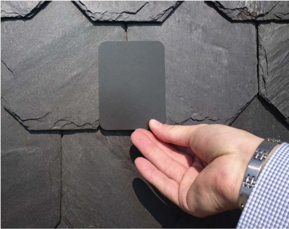
Material in Direct Sun compared to existing slate roof
