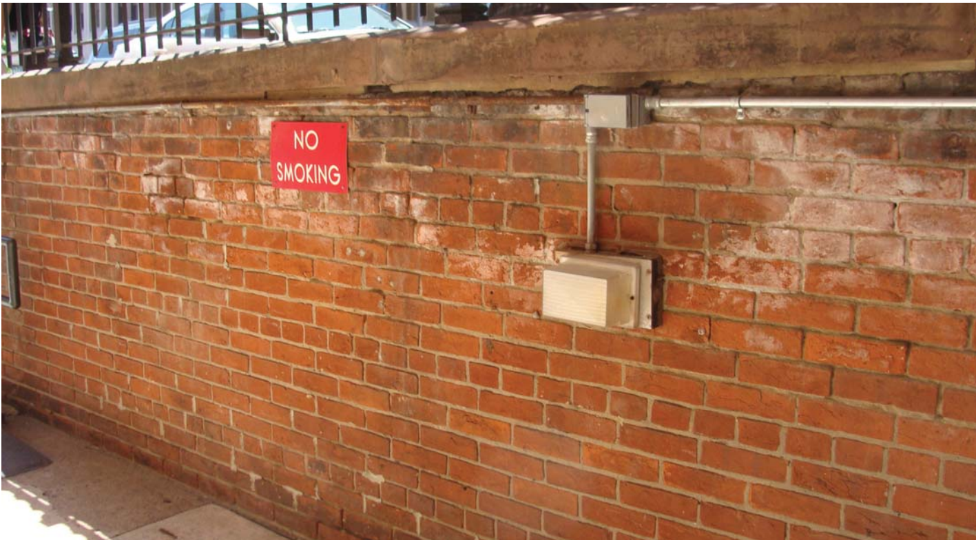
Lighting fixtures and conduit throughout moat to be replaced
