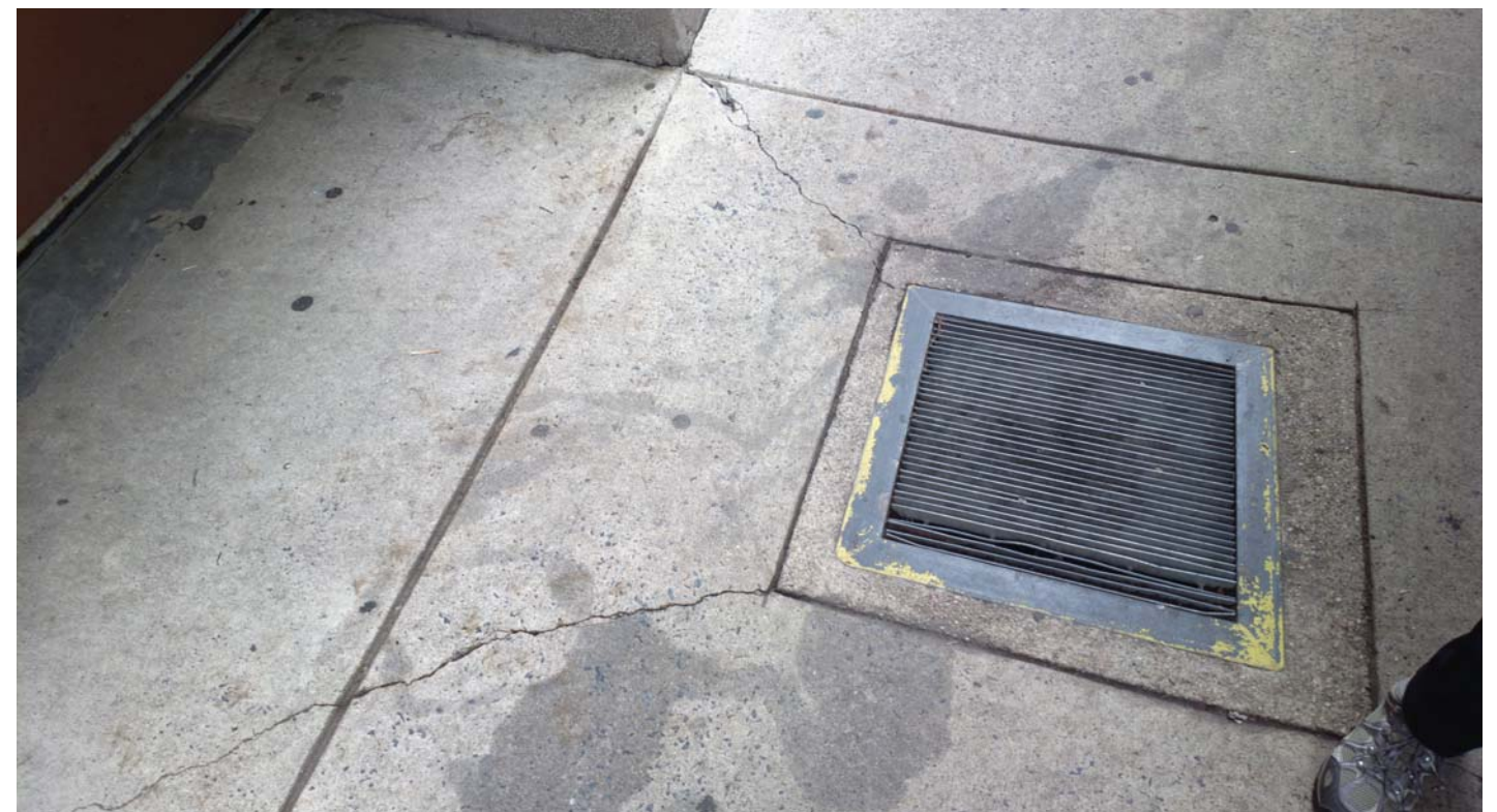
Deteriorated moat slab
