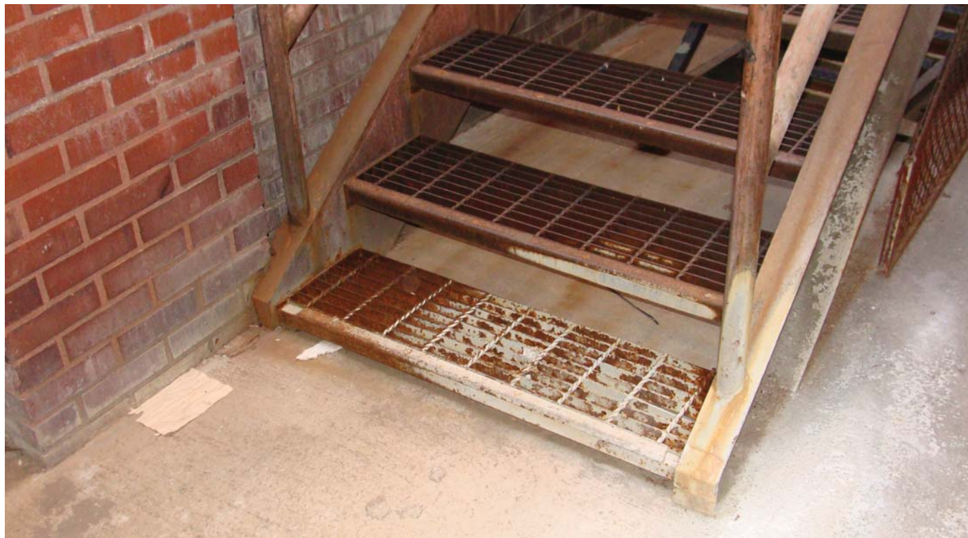
View of non-compliant stair treads
