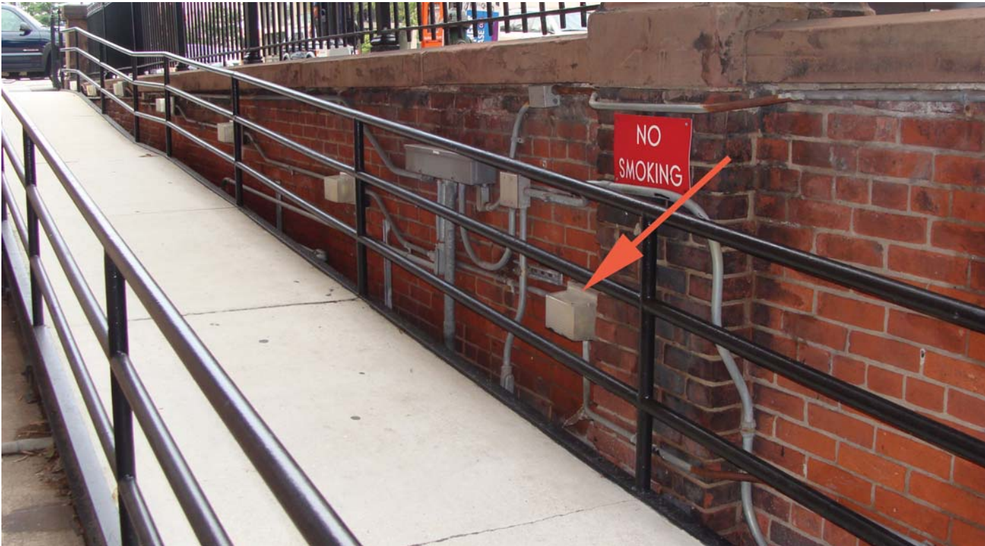
Lighting fixtures and conduit at ramp to be replaced
