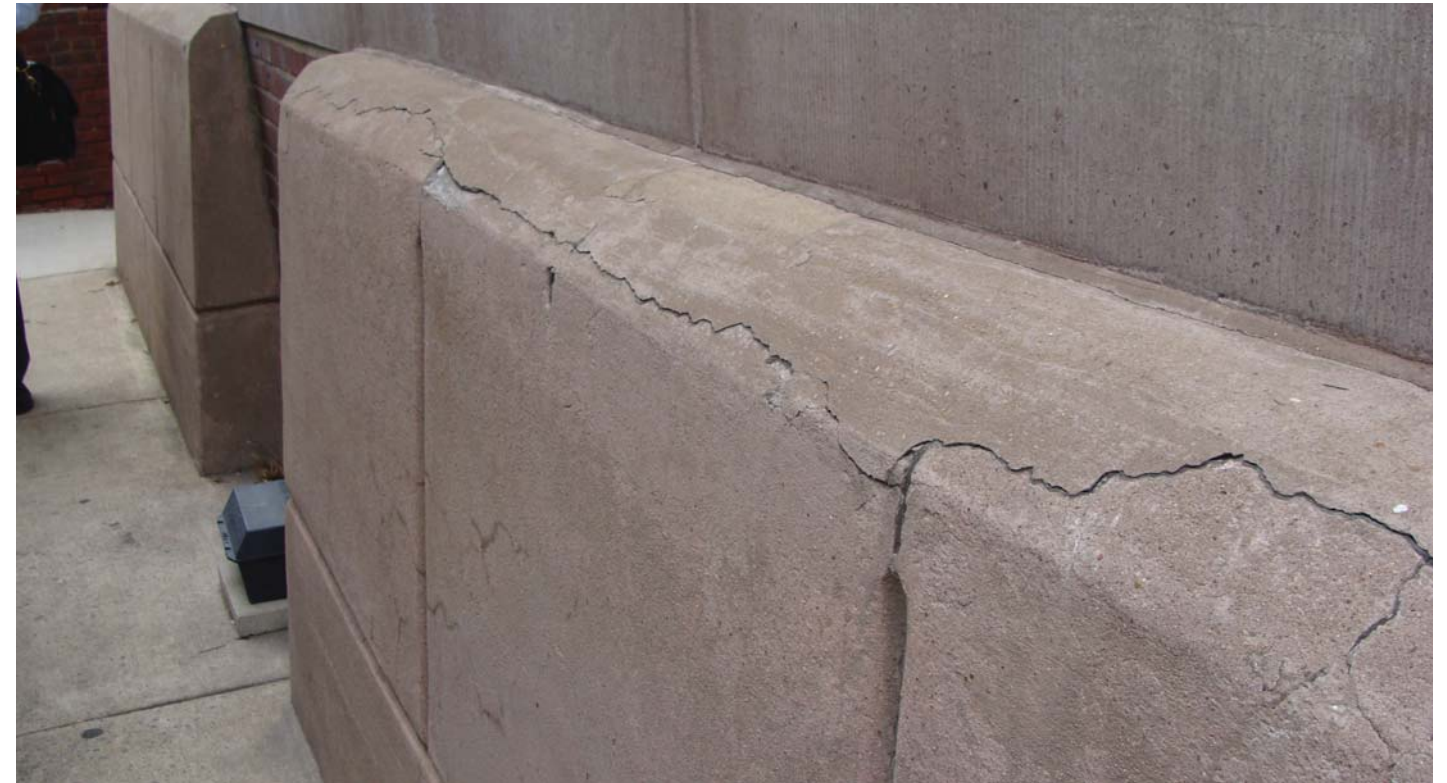
Deteriorated cementitious stucco at areaway
