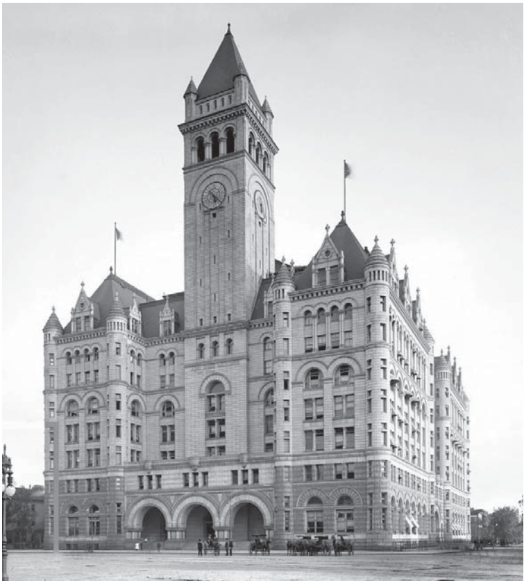
Historic North elevation
