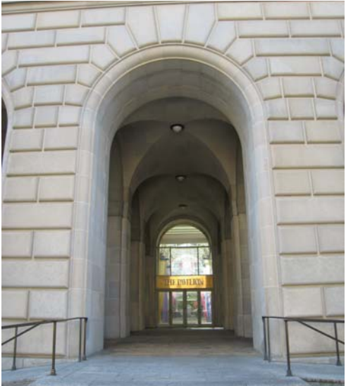
Existing view through entrance arcade
