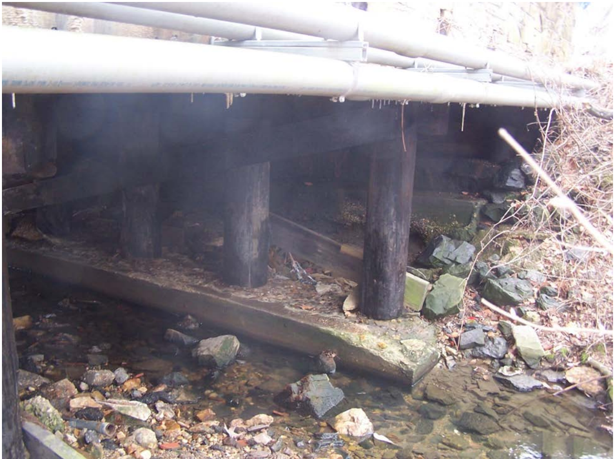
Figure 3: North Drive Bridge Substructure
