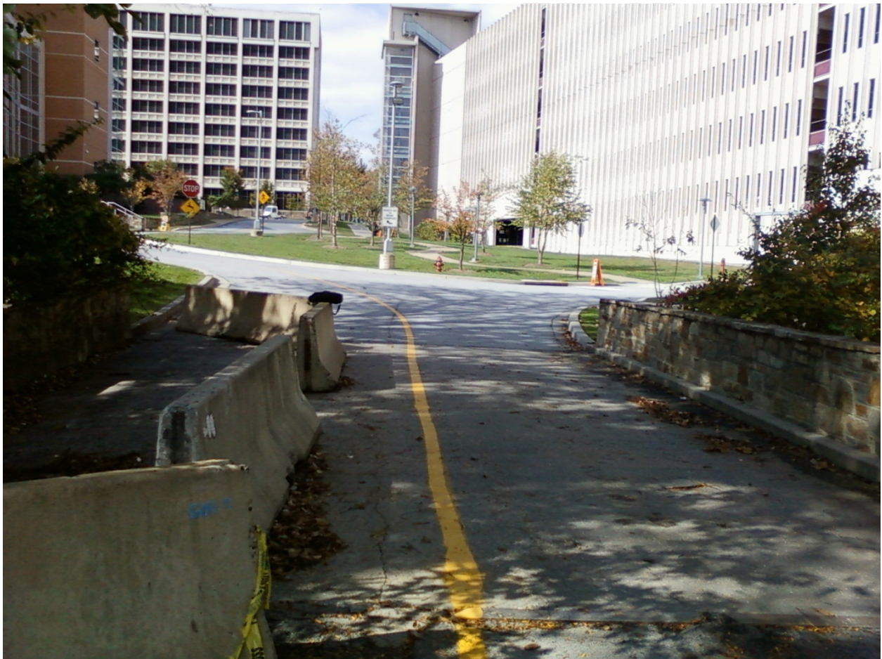
Figure 2: North Drive Bridge partial closure
