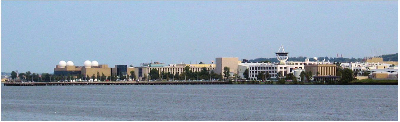
A panoramic view of the NRL from the Potomac River shows the dense urban environment and flat topography along the Potomac River waterfront. Source NRL.
