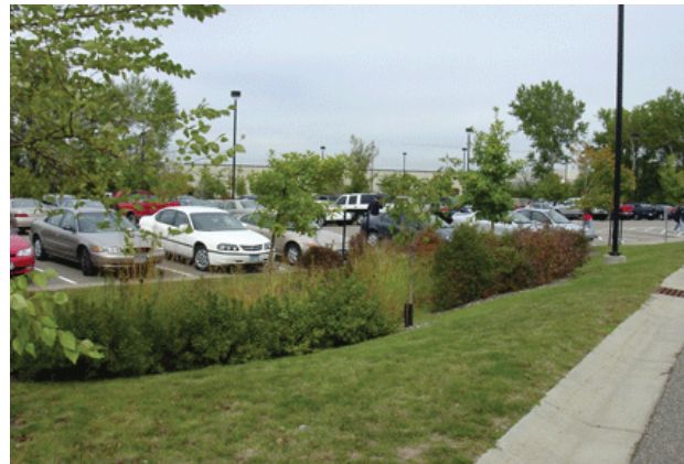
Bioretention swales can filter stormwater runoff and prevent erosion.
