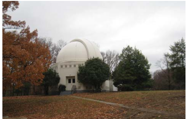
Building 39, the Equatorial Telescope Laboratory, supports the USNO's RDT&E mission.
