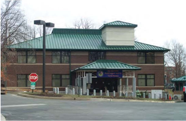
Building 56 depicts the natural brick color and green roof color scheme used in other facilities on the Installation.
