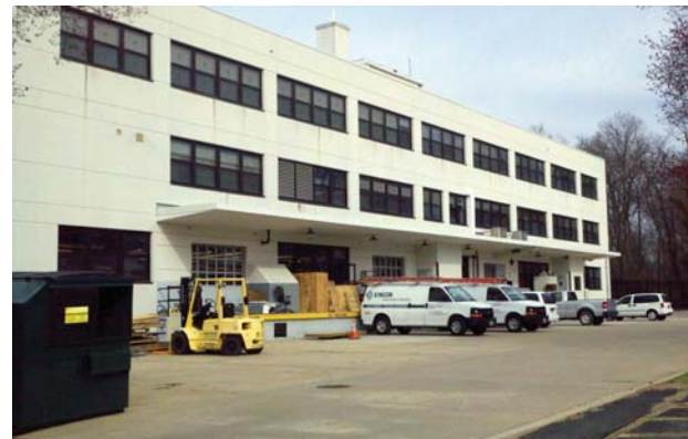
Building 52 is among the tallest structures, with three stories.
