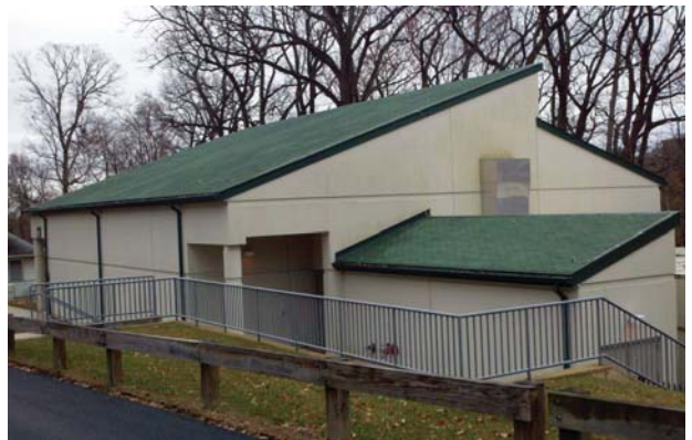
Building 50 houses the Atomic Clock, an integral mission at NSF Naval Observatory.
