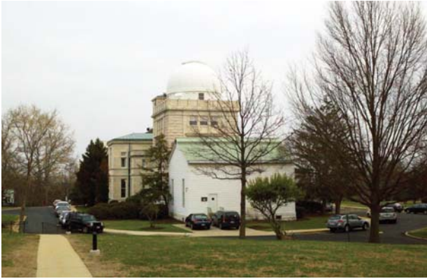
Several facilities on NSF Naval Observatory are within the minimum AT/FP setback from roadways and parking.
