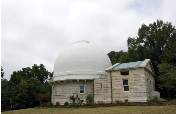
Building 2, the Great Equatorial/26-inch Telescope Building, considered a contributing NRHP building.
