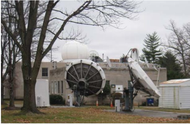
Building 78 houses the Simon Newcomb Laboratory.
