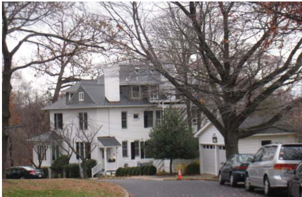
Building 61 is the only temporary lodging facility on NSF Naval Observatory.
