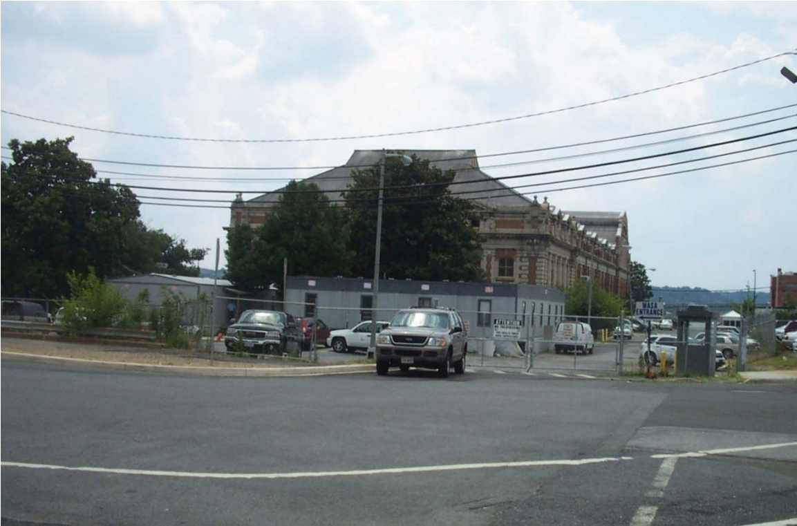
Looking South towards Main Pumping Station from NJ Avenue
