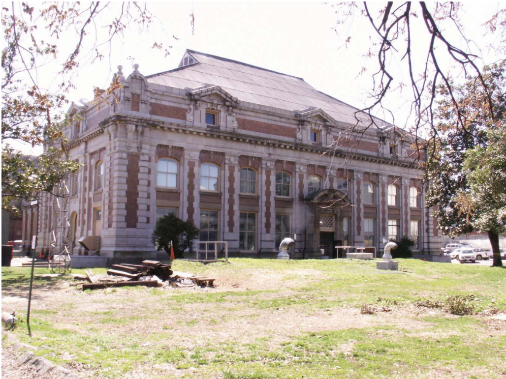
Looking Southwest Inside DC Water Fence
