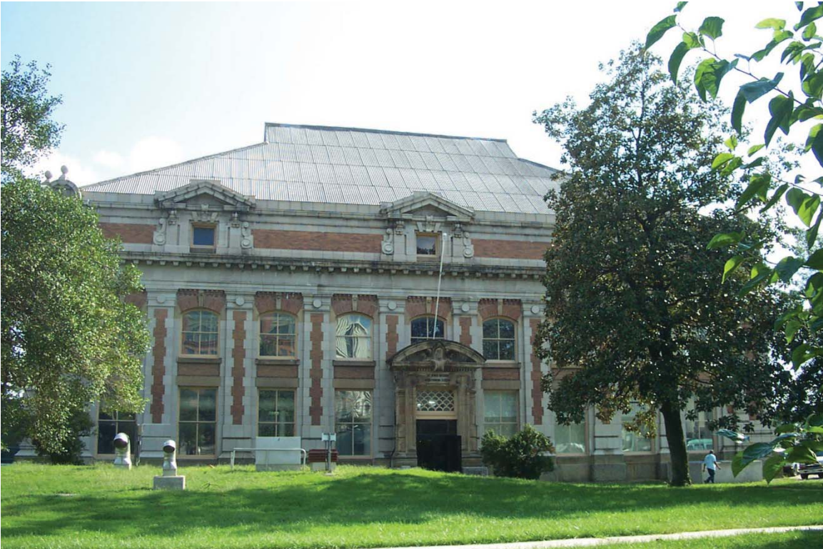
Looking South inside DC Water Fence
