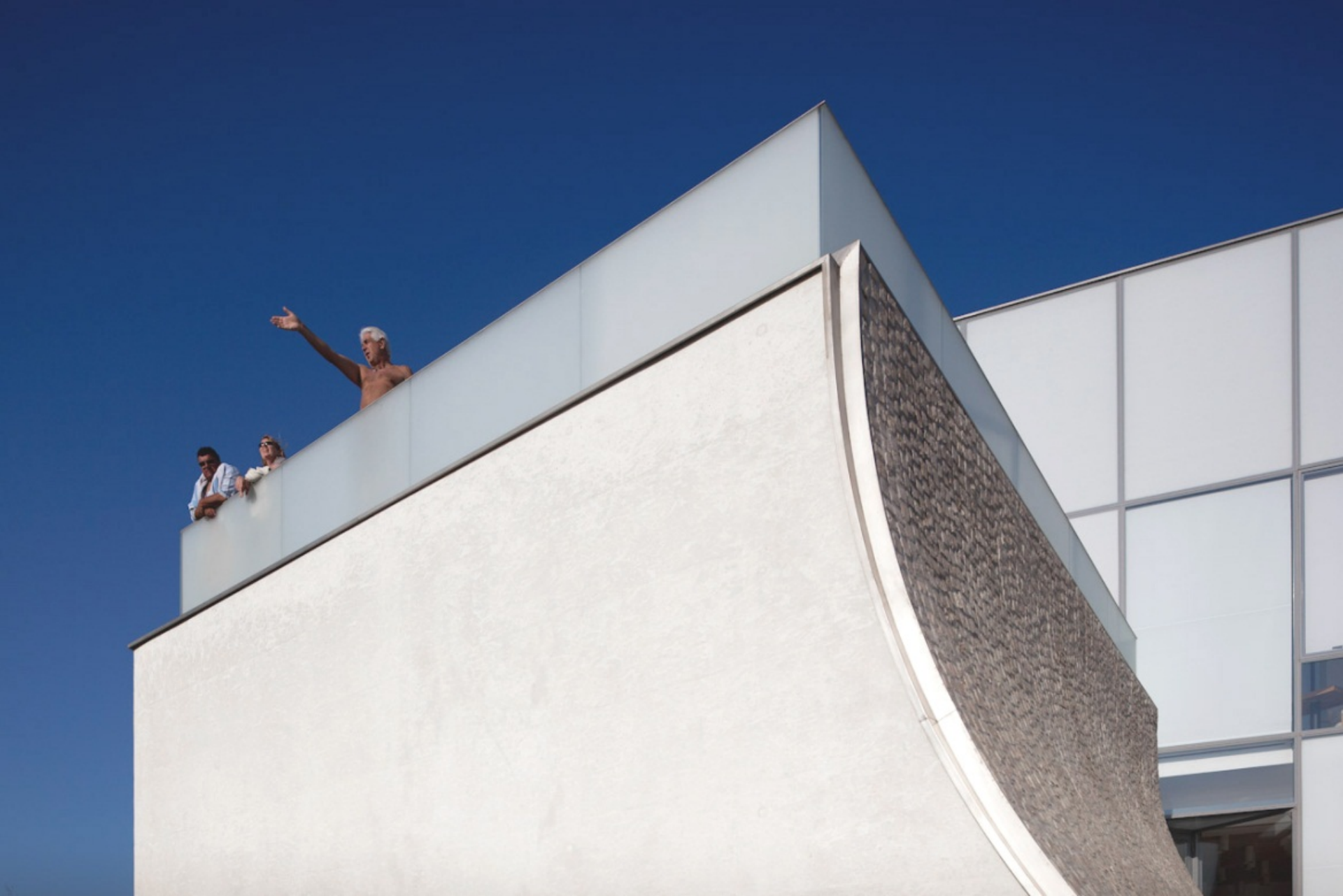
CITE DE L'OCEAN ET DU SURF BY STEVEN HOLL ARCHITECTS EXAMPLE OF WHITE CONCRETE AND TRANSLUCENT GLASS
