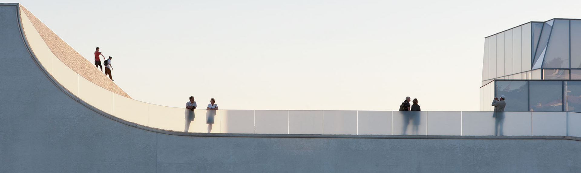
CITE DE L'OCEAN ET DU SURF BY STEVEN HOLL ARCHITECTS EXAMPLE OF WHITE CONCRETE AND TRANSLUCENT GLASS
