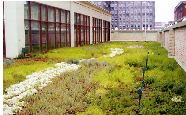
Installation of a green roof will reduce stormwater runoff and improve water quality
