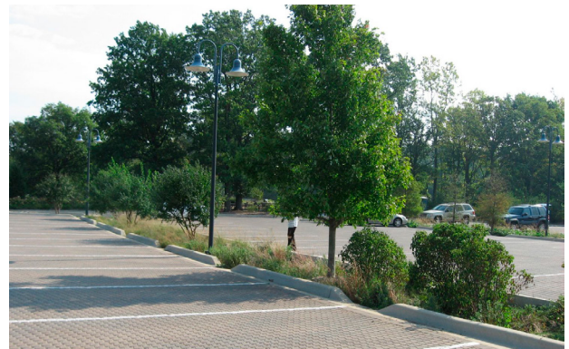
Example of a parking lot designed with permeable pavers and rain garden
