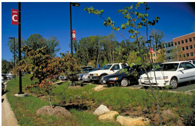
An example of creating bioretention areas within and at the perimeter of parking lots for stormwater management
