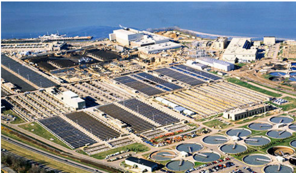
The DC Water Blue Plains AWTP, located just south of JBAB, treats wastewater from the installation
