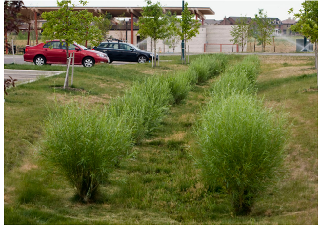
Vegetated bioswales along roadways help manage and treat stormwater runoff
