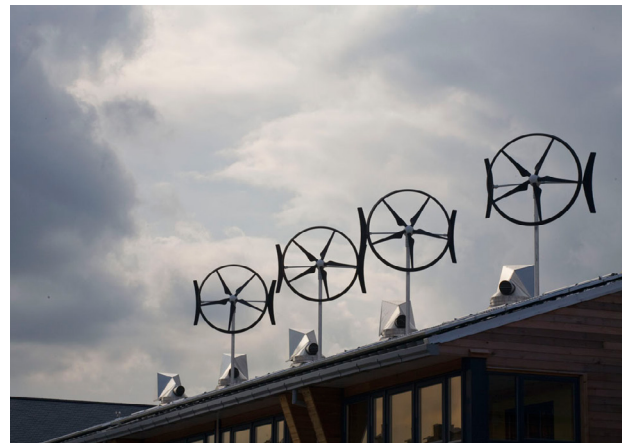
Wind turbines are NOT recommended for renewable energy production at JBAB due to height restrictions and low wind speed in the region
