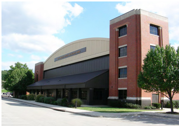
Hangar 2 is the practice facility for the U.S. Air Force Band
