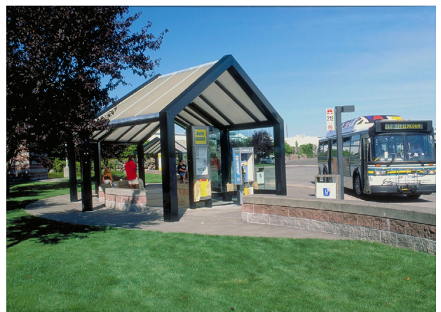
Safe and comfortable transit facilities makes alternative transportation a viable option for users
