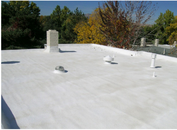
The use of cool roof materials helps reduce the solar heat absorption of buildings
