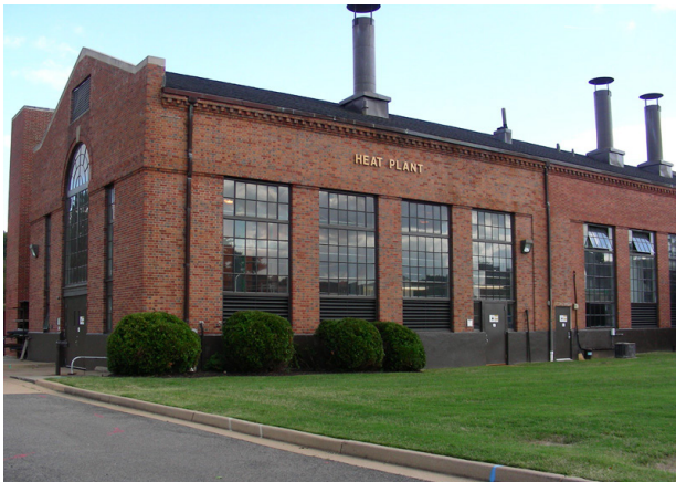
Building 18 provides heating and cooling
