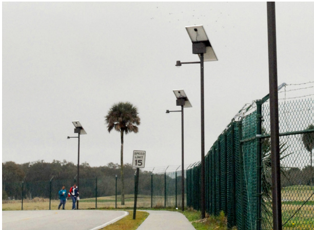
Installation of solar-powered LED street lights will cut down energy consumption
