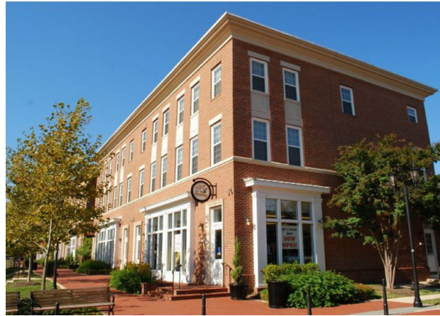
The public and private partnership strategy employed by Fort Belvoir helped with the creation of the installation's mixed-use town center
