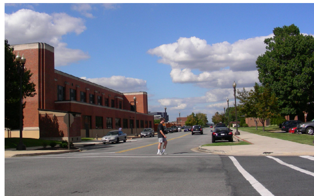
Sidewalks and crosswalks are provided throughout the residential and administrative areas on the Bolling side
