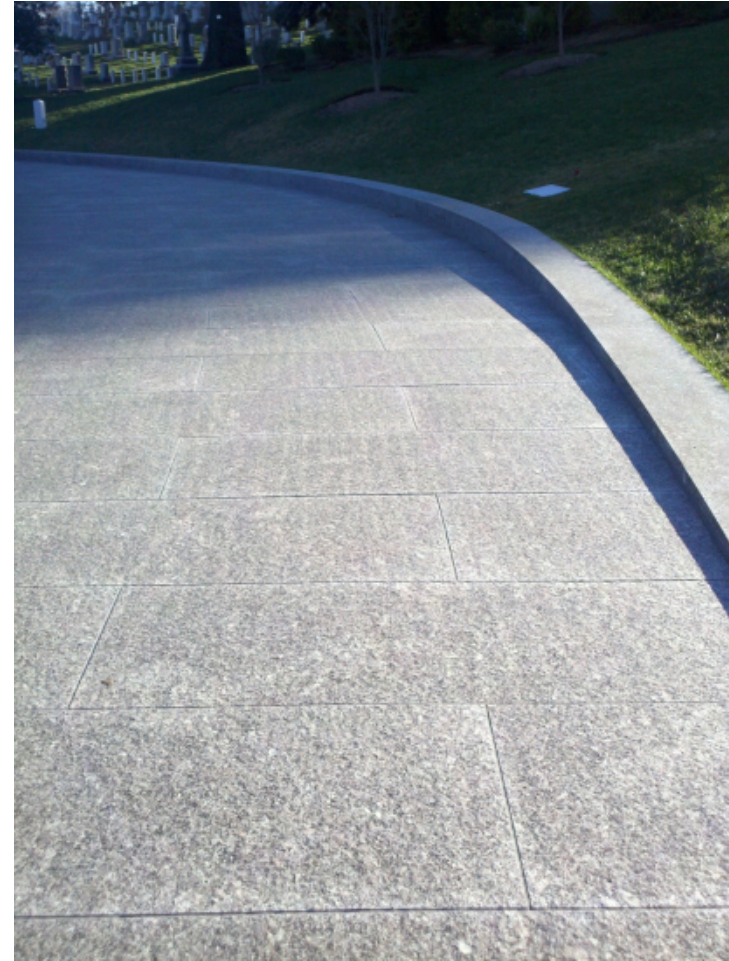
Existing granite walkway at Arlington National Cemetery
