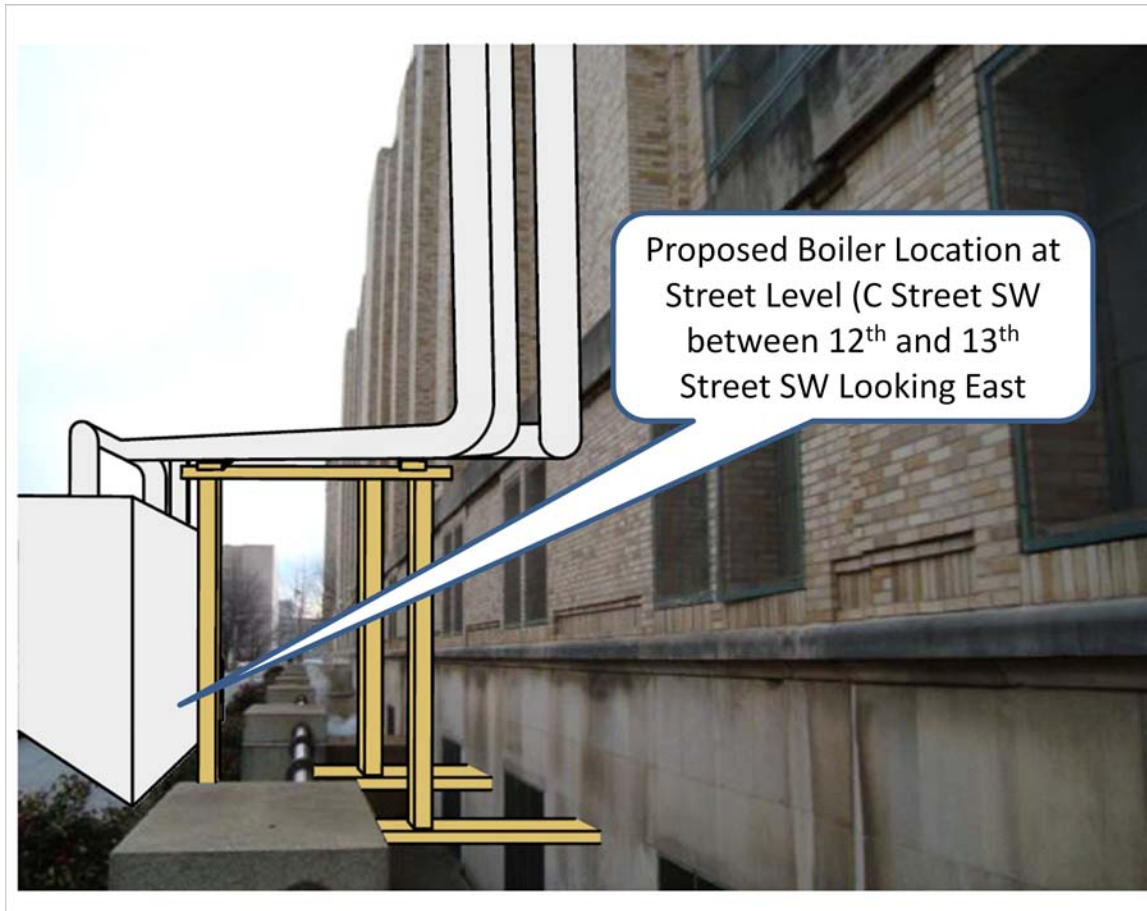
Figure 11 - North Elevation Photo Showing Proposed Boiler Location
