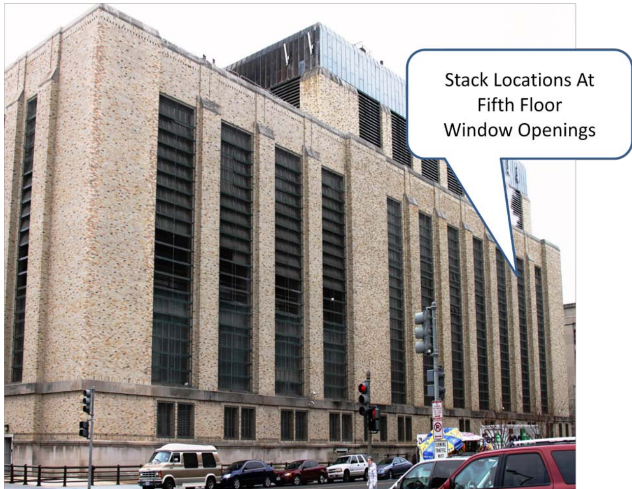
Figure 7 North Elevation Photo Looking West
