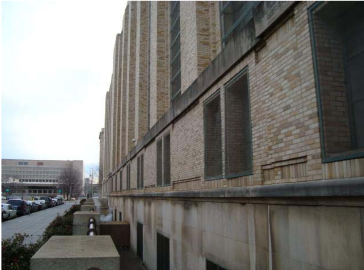
Figure 10 - North Elevation Photo Looking East
