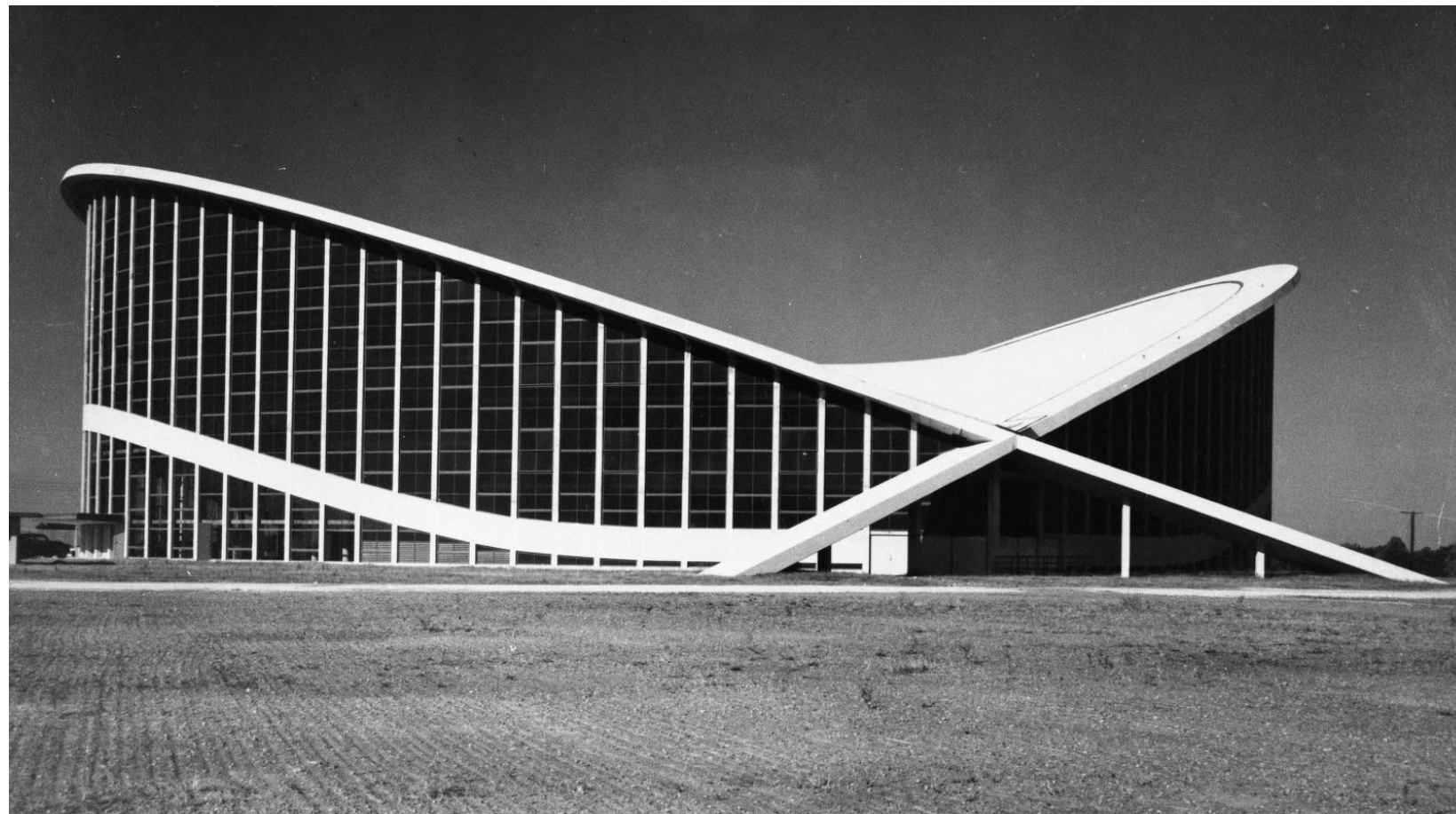
1952 - Dorton Arena; Hyperbolic Paraboloid Dome
