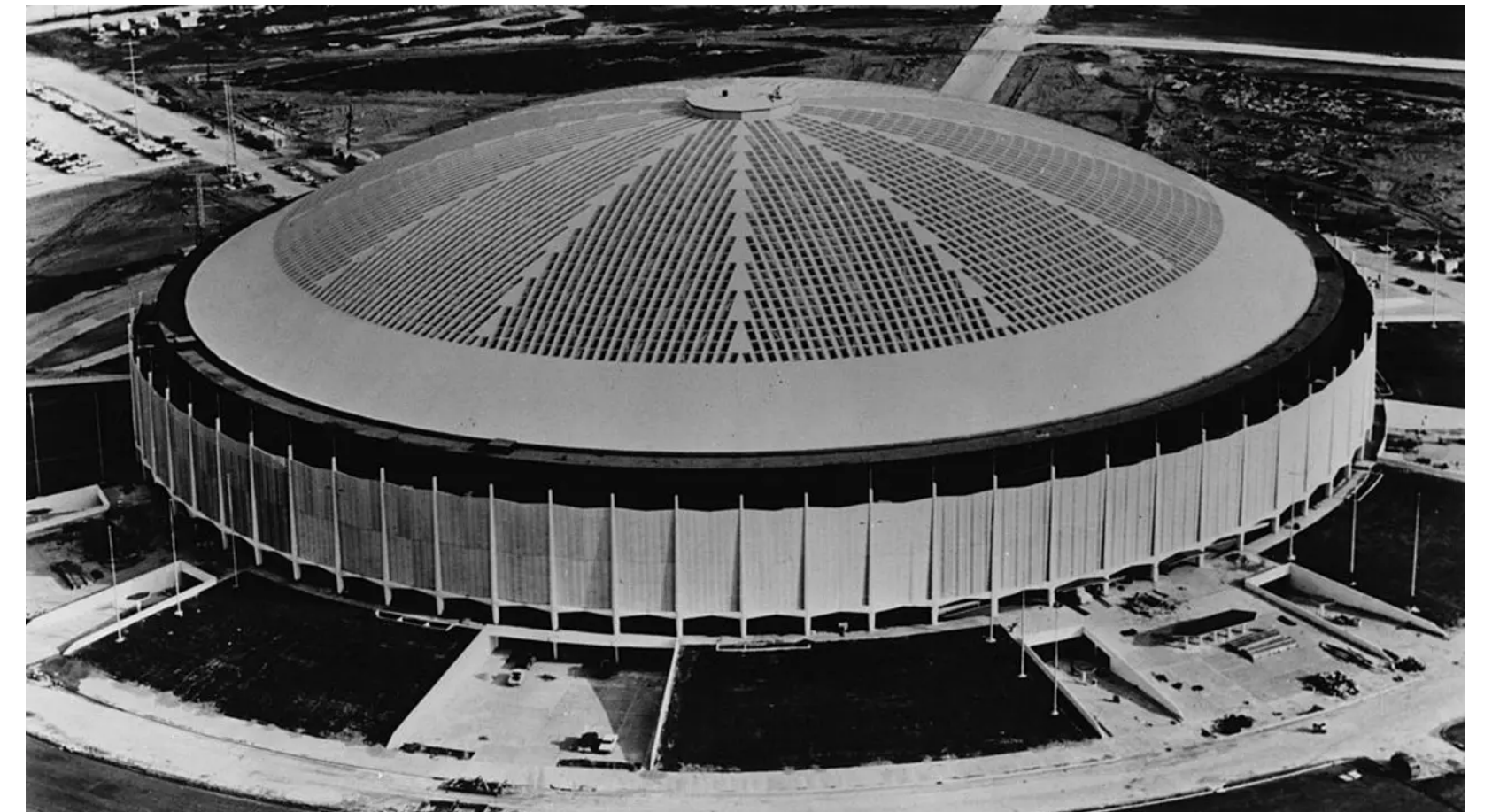
1964 - Houston Astrodome; Steel Lamella Dome
