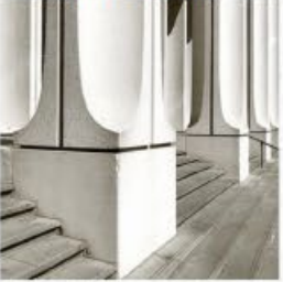
C.I.P. CONCRETE STRUCTURE
