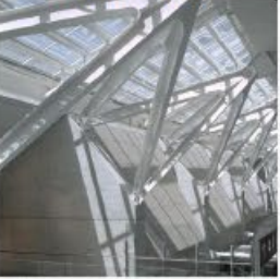
BUILT-UP STEEL STRUCTURE
