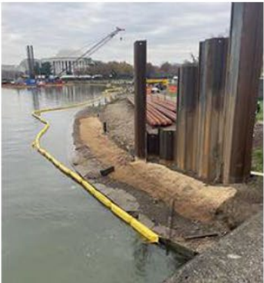
Image shows construction at the seawall south of the Inlet bridge.
