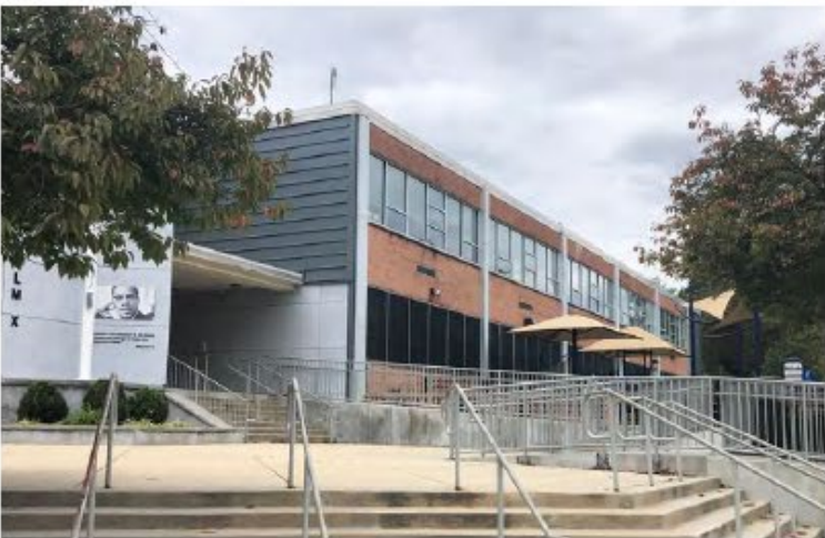
East Wing Elevation from Mississippi Avenue Entrance
