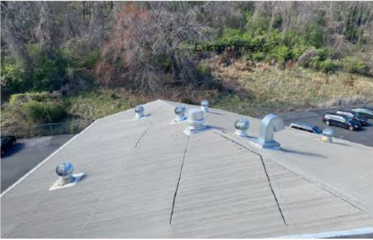
Site to North from Roof
