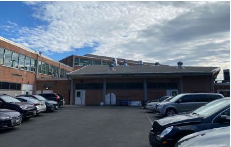
Cafeteria Northeast Elevation
