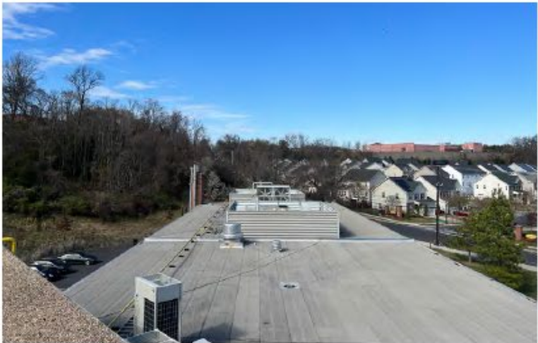
East Wing Roof
