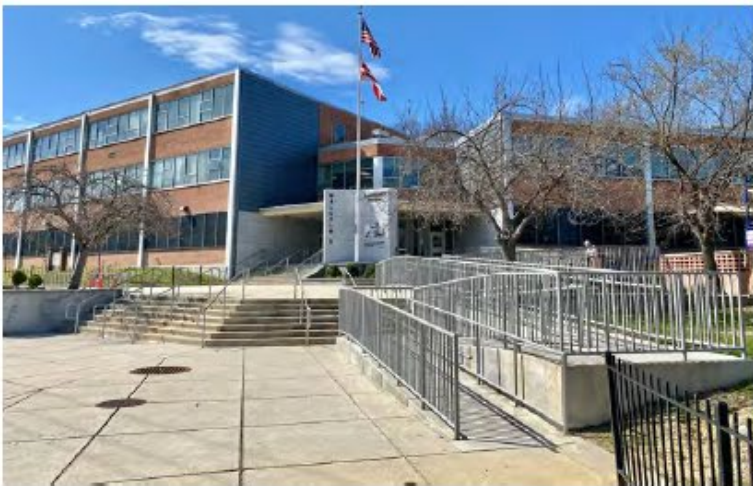
Main Building Entrance from Mississippi Avenue
