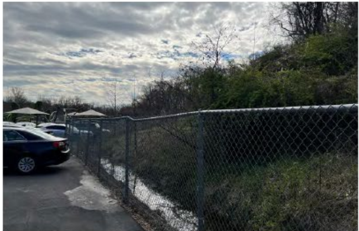
North Hillside and Site Gutter
