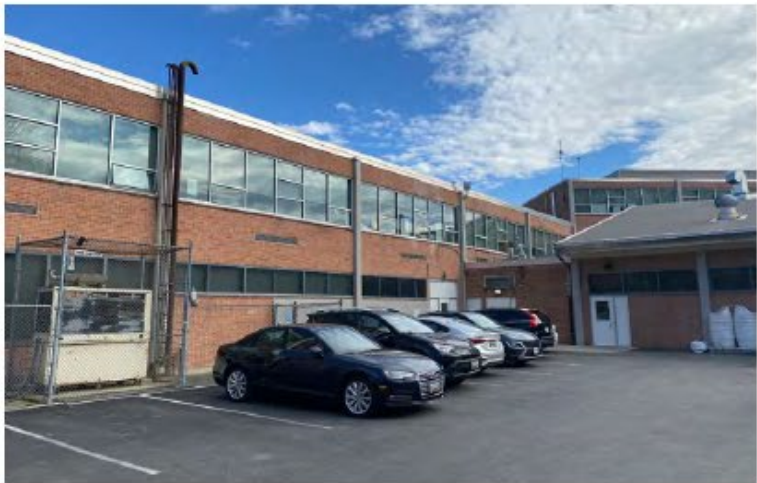
East Wing Rear Elevation
