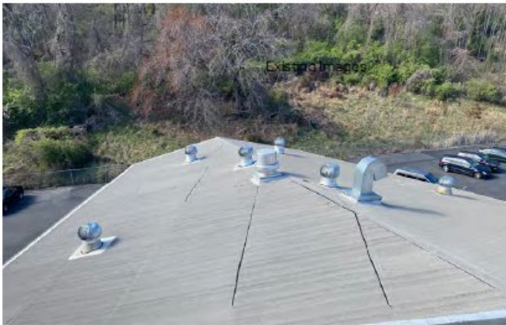
Site to North from Roof
