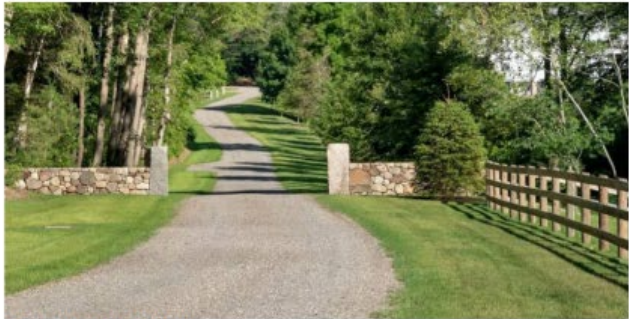
Crushed Stone Paving
