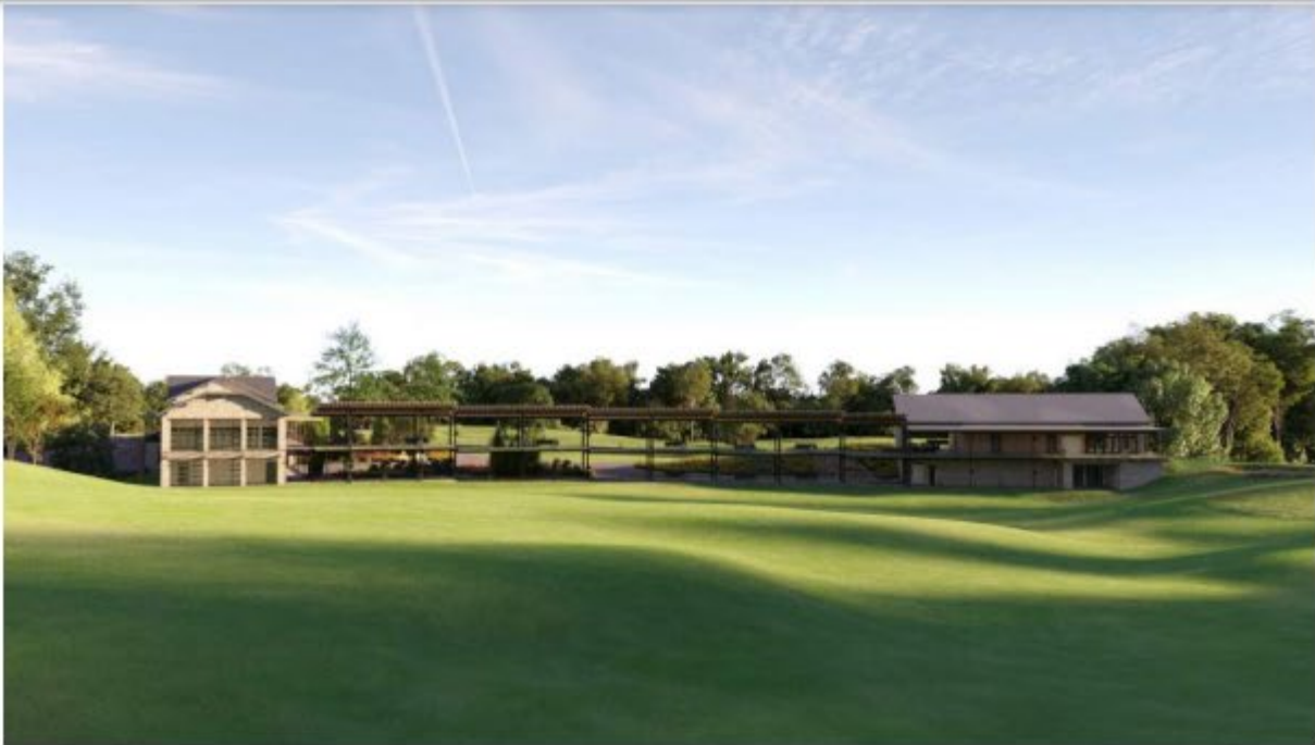
VIEW LOOKING SOUTHWEST FROM TOP OF DRIVING RANGE
