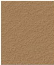
Painted Stucco (Side Walls)
