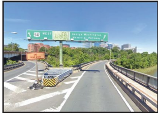
Existing cantilever sign structure (I-66 WB ramp to GW Parkway/ Highway 50)
