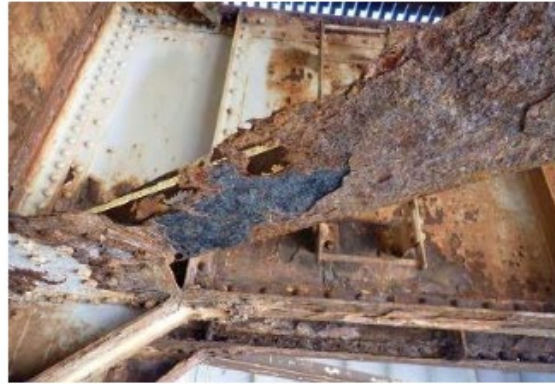
Large holes in lateral bracing
