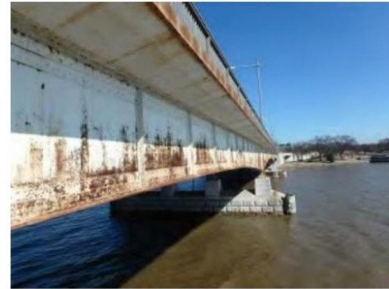
Corroded steel
