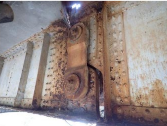
Corrosion at pin and hangar
