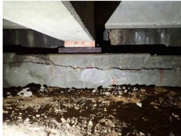
Crack in abutment
