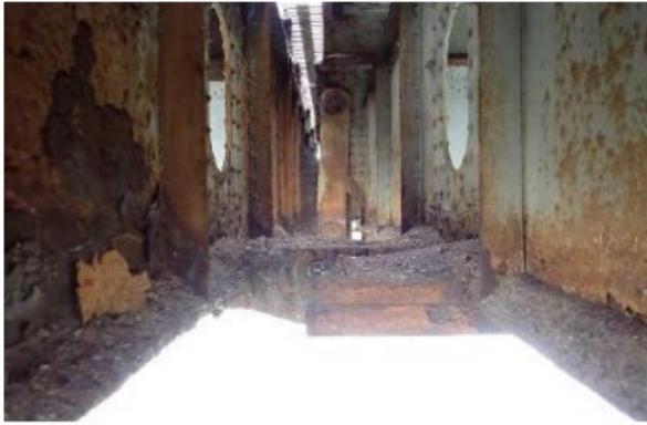
Typical debris on bottom flanges of floorbeams and girders at the finger joint
