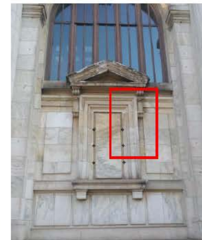
Anchor points in grout joints
