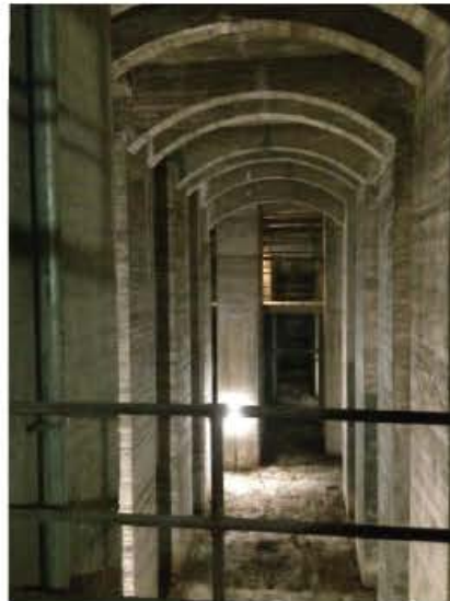
5 - VIEW INTO THE STATUARY CHAMBER UNDERCROFT FROM THE MEZZANINE
