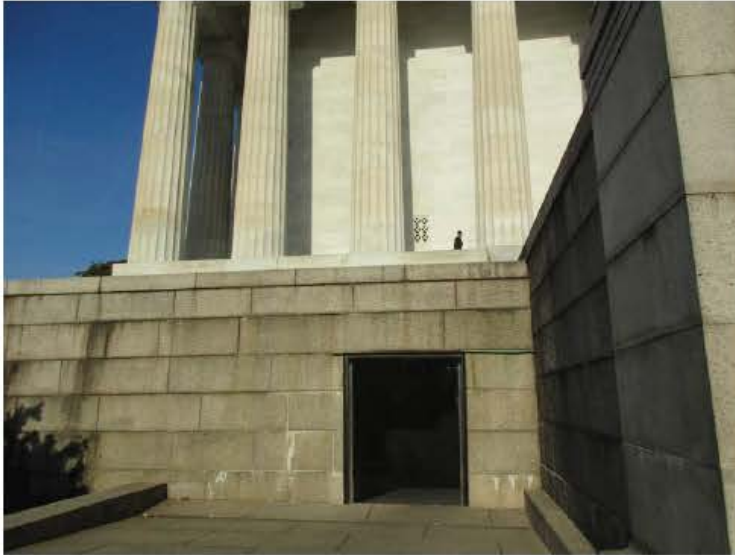
1 - SOUTH UNDERCROFT DOOR
