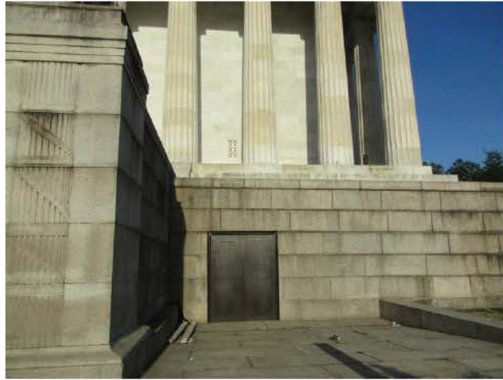
2 - NORTH UNDERCROFT DOOR
