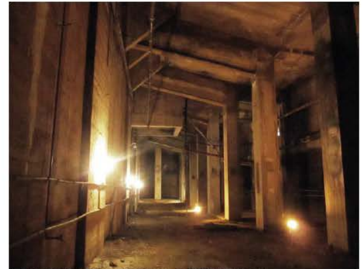
6 - VIEW OF THE RAISED TERRACE UNDERCROFT
