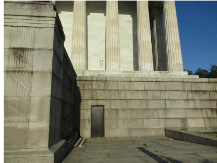
2 - NORTH UNDERCROFT DOOR
