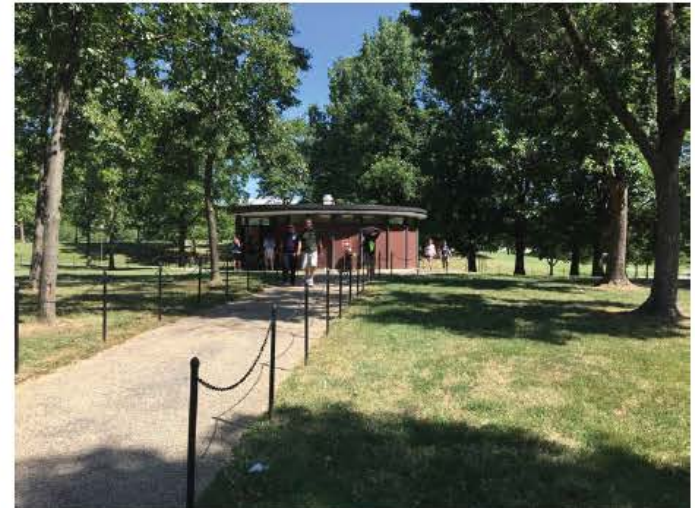
5 - CLOSEST PUBLIC RESTROOM
