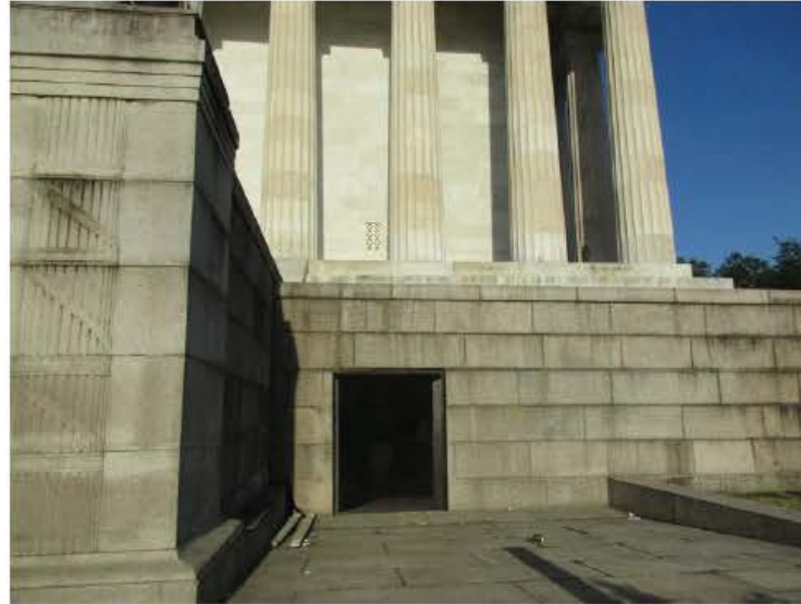
2 - NORTH UNDERCROFT DOOR
