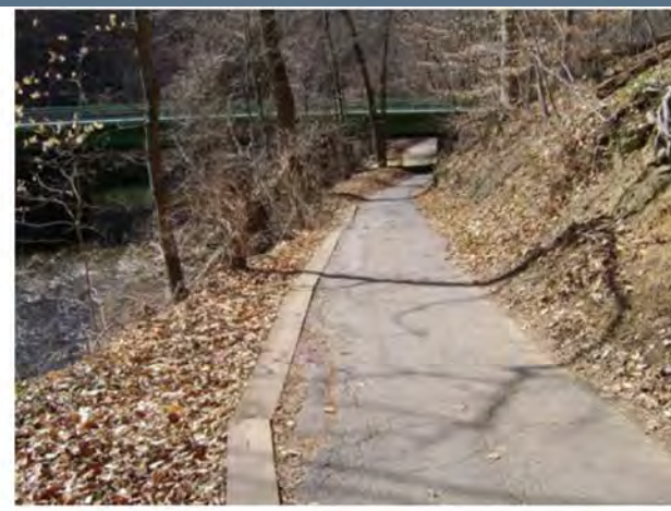
Existing Timber Edge Support
