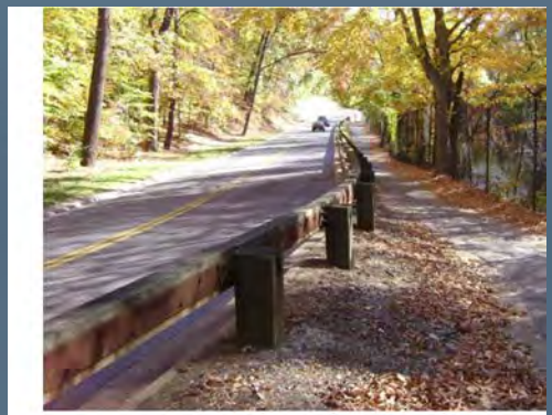
Existing Timber Steel Backed Timber Barrier
