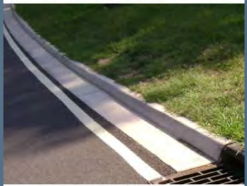
Existing Concrete Curb and Gutter
