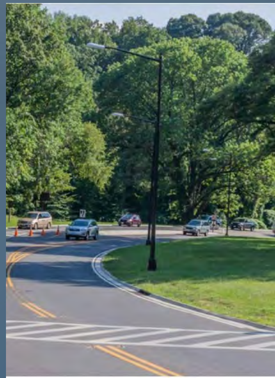
Existing Cobrahead Lighting
