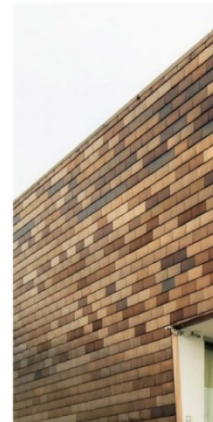
Metal Tile - Lapped Shingle Installation
