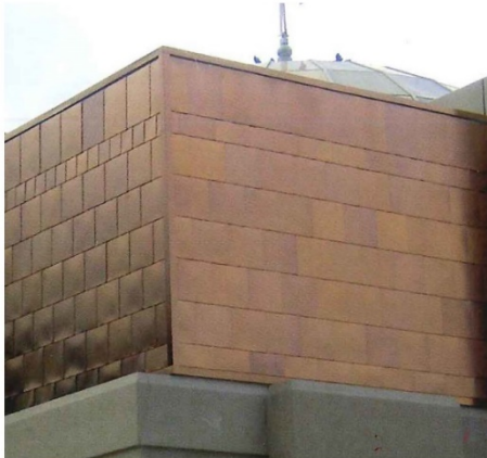
Metal Panel - Flat Lock Installation
