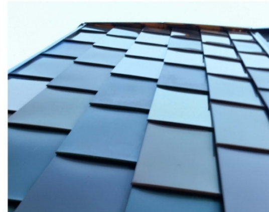
Metal Panel - Flat Lock Installation
