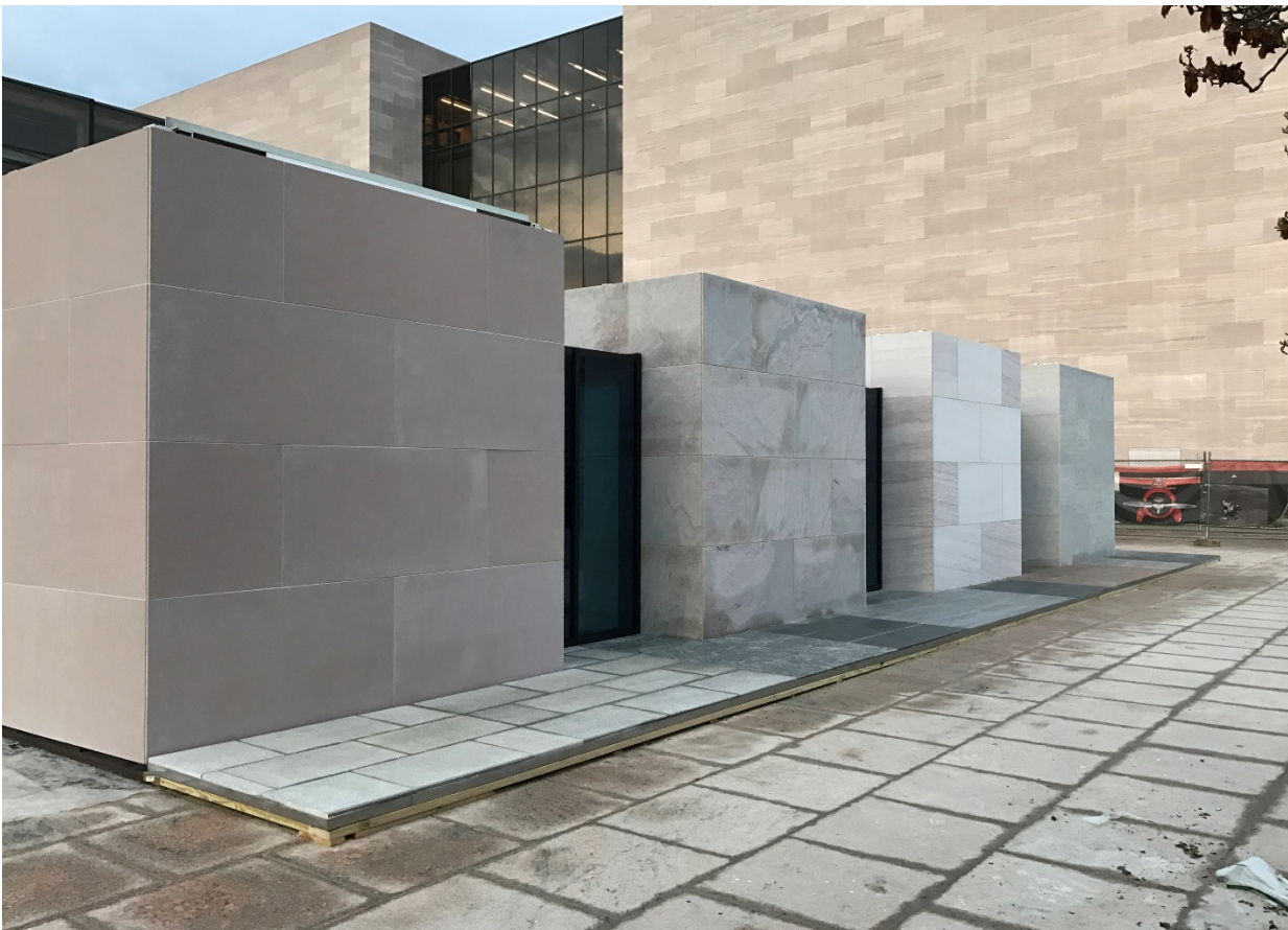
Mockup of the four cladding options under consideration constructed on the northeast corner of the NASM terrace, showing from left to right Ultra High Performance Concrete (UHPC), Echo Lake granite, Tennessee Pink marble and Saint Claire limestone.
