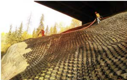
Geo-cell reinforcement with soil and plants
