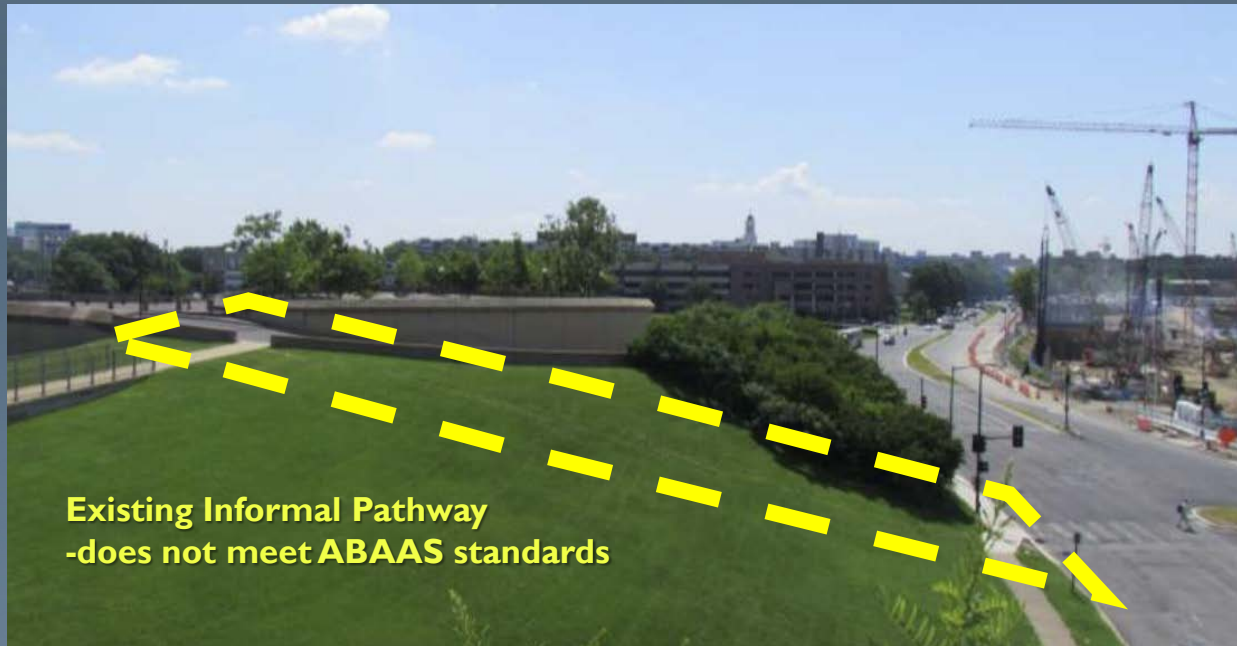
View of Banneker Park from the Case pedestrian bridge
