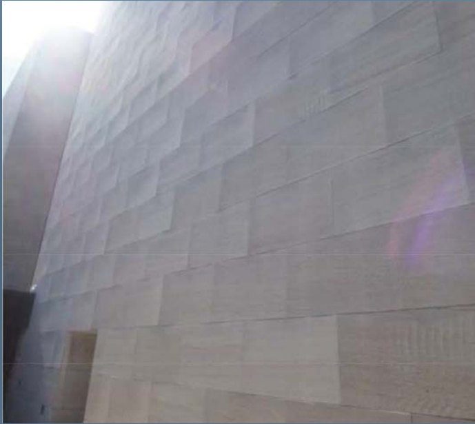
Warped Stone Panels on North Facade
