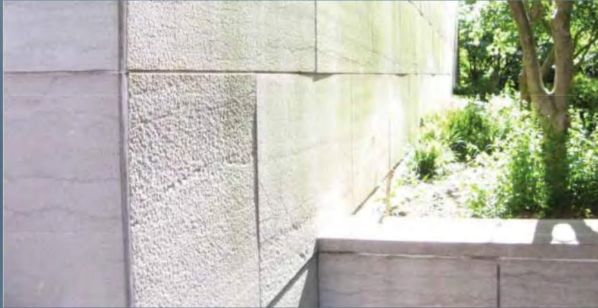
Warped Stone Panels on West Facade
