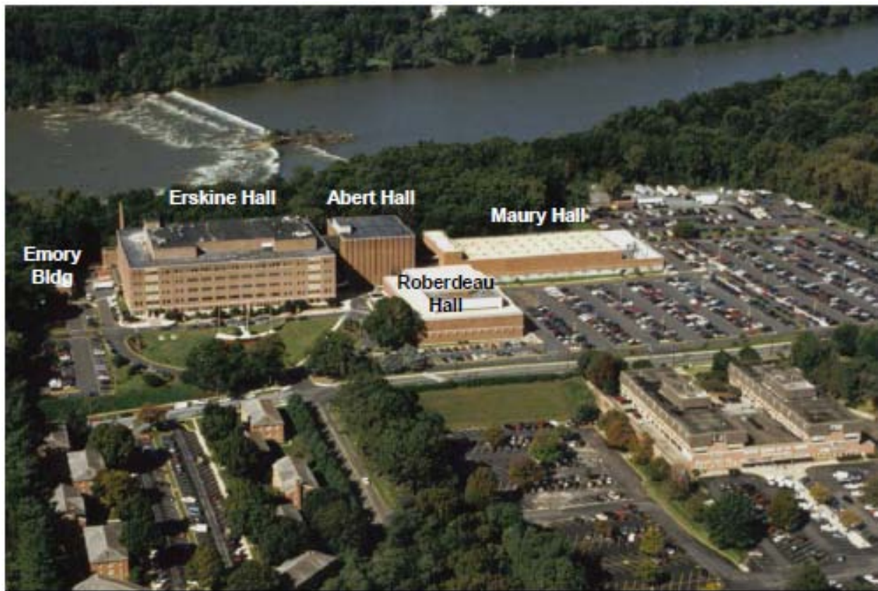
Birdseye view of the existing condition of the installation, looking west (the installation fronts Sangamore Road, which runs through the center of the photograph)
