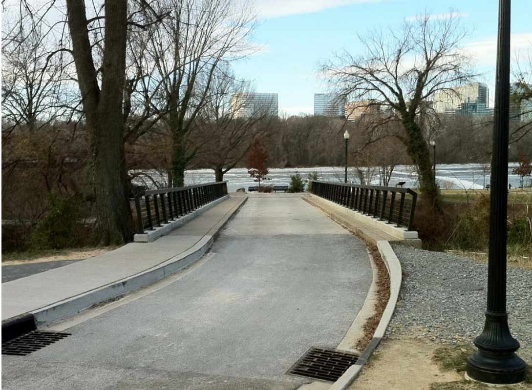
New condition of the bridge over Rock Creek (looking towards the Potomac River)
