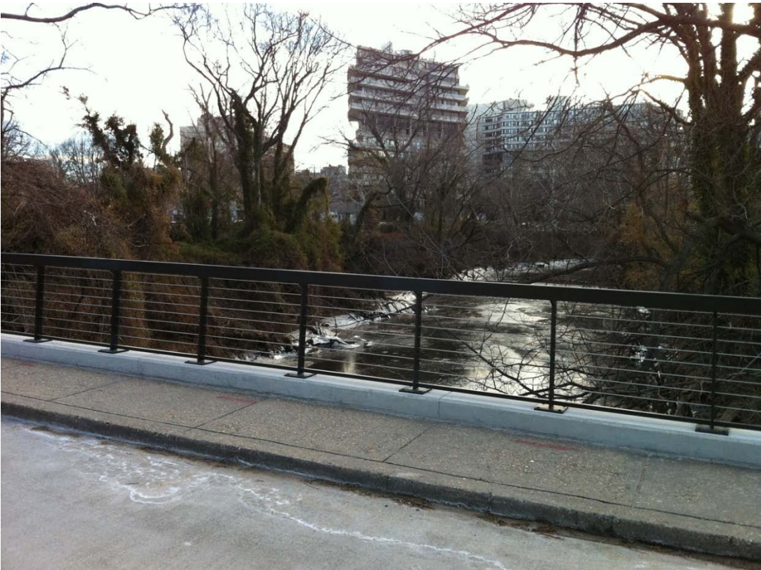
New condition of the bridge over Rock Creek, showing the new railing (looking east)
