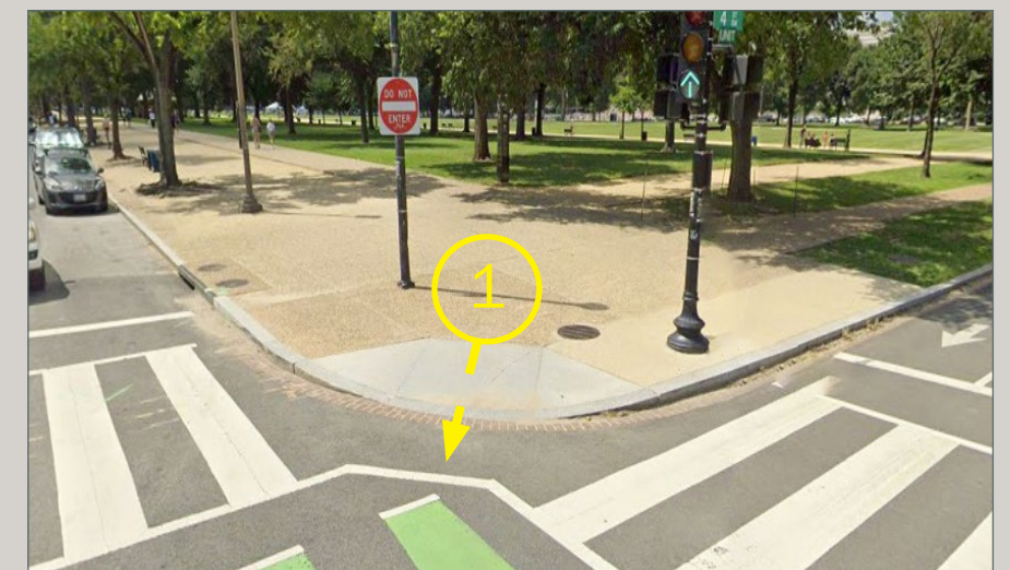
Figure P-14: Do not use one blended transition curb ramp oriented towards the middle of an intersection, unless specifically designed as a Barnes-Dance intersection. 34
