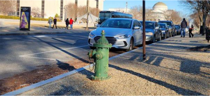
Figure FH-1: Green fire hydrants signal that the hydrant is operational. Black hydrants signage the fire hydrant is not operational.
