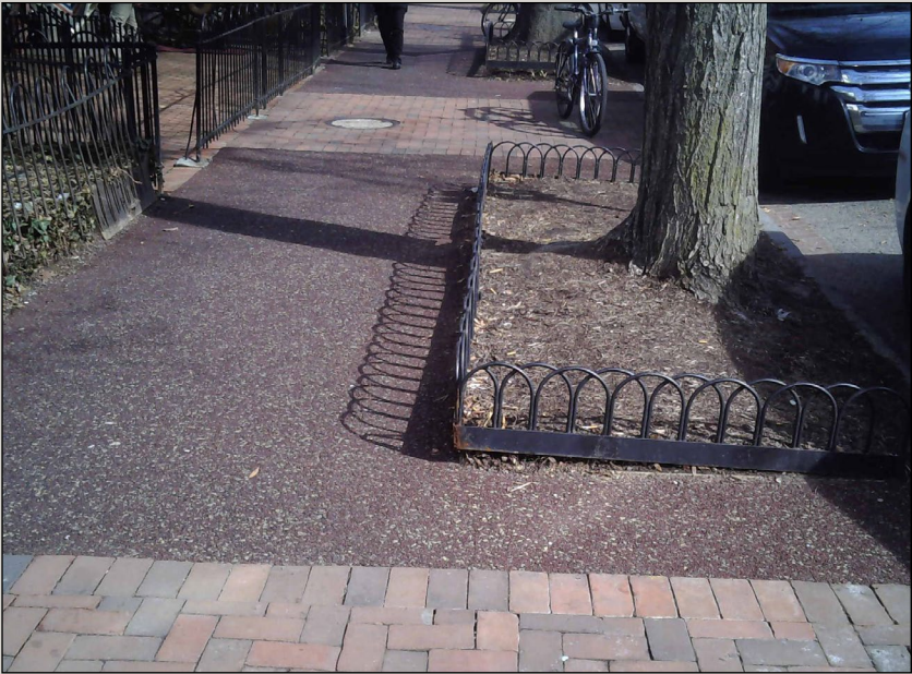
Figure T-7: Appropriate installation of flexible porous pavement within the Capitol Hill Historic District near Eastern Market.
