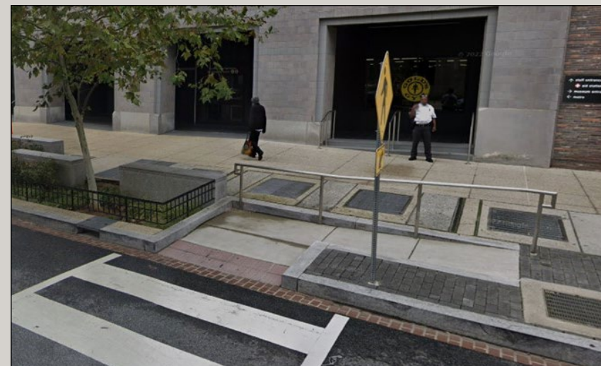
Figure SM-5: Green Infrastructure planter with universally accessible mid-block circulation ramp connecting the curb to the sidewalk along D Street, SW between 3rd and 4th Streets.
