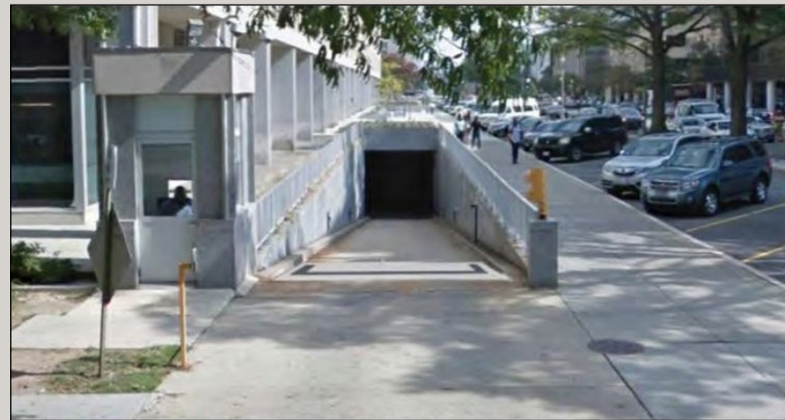
Figure PC-2: Beam barriers are an alternative to more intrusive wedge vehicular barriers and higher-maintenance retractable bollards.
