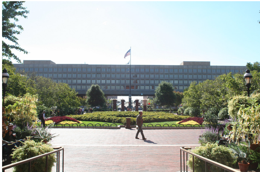
VIEW 2 EXISTING CONDITIONS
