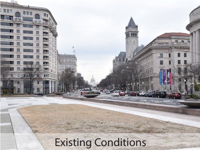
View from SE corner of Freedom Plaza, looking southeast (Viewshed Analysis View 9)
