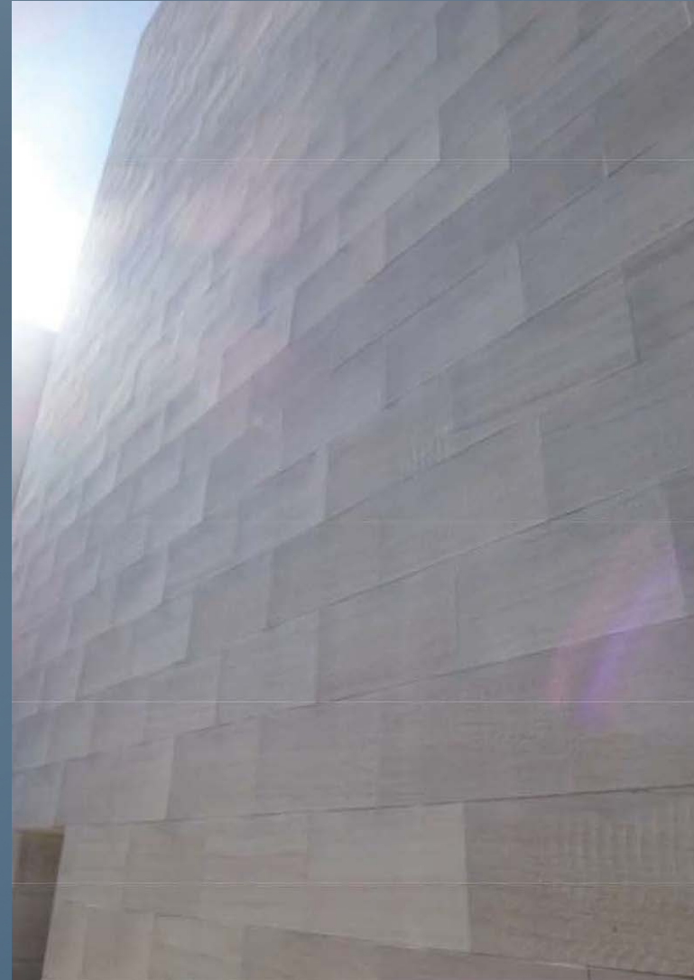
Existing warped and cracked Tennessee Pink
