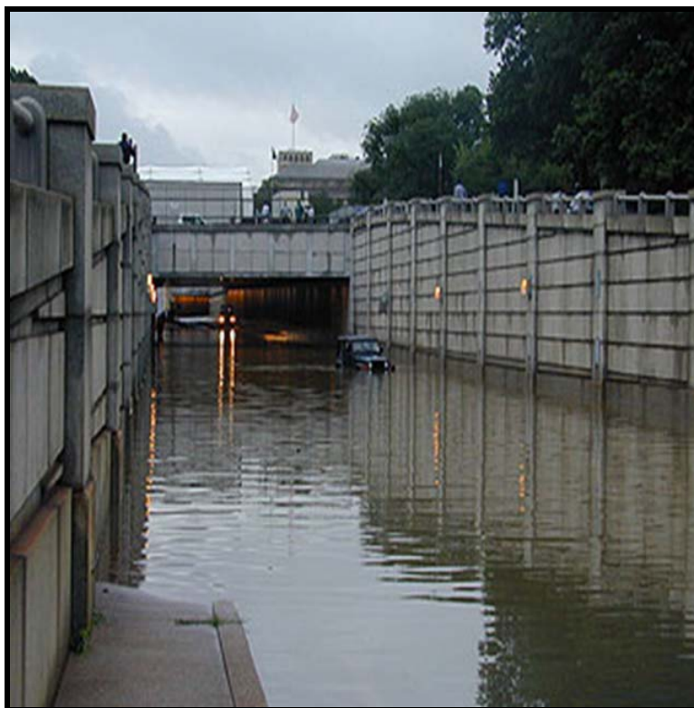
Location: 12 th Street Tunnel Source: NCPD
