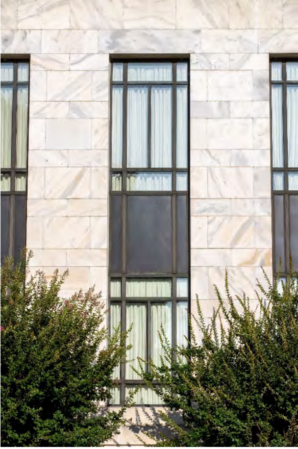
DOUBLE HEIGHT BRONZE WINDOWS W/ ALBERENE STONE SPANDREL PANELS
