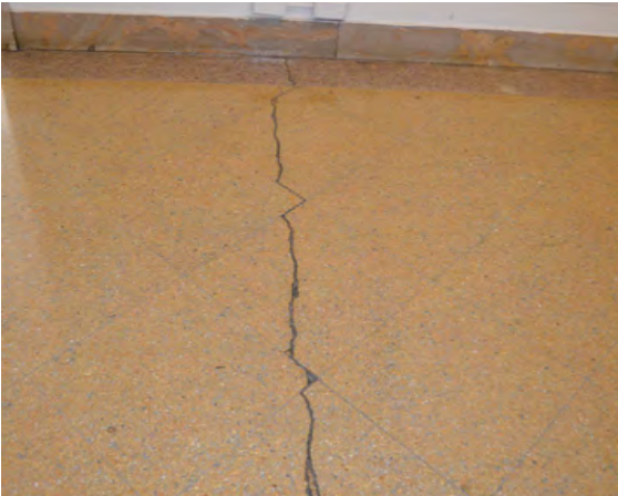
Terrazzo Flooring (Localized areas of cracking and previous repairs)
