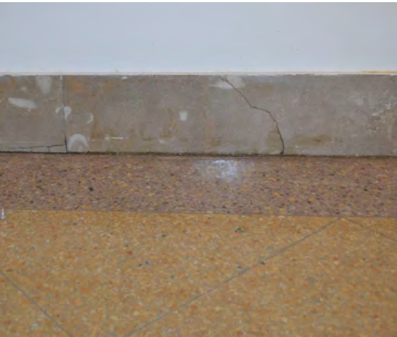
Marble Wall Base (Localized areas of cracking)
