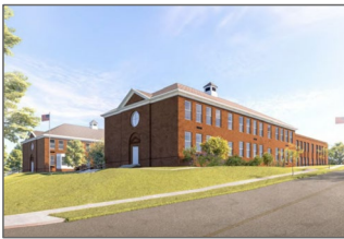
(4.) Bunker Hill Elementary
