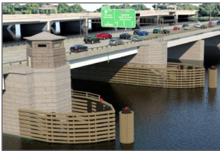
(4.) Arland D. Williams Jr. Memorial Bridge Span Replacement
