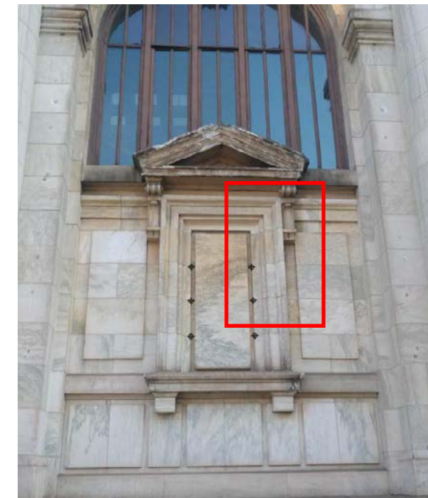
Anchor points in grout joints
