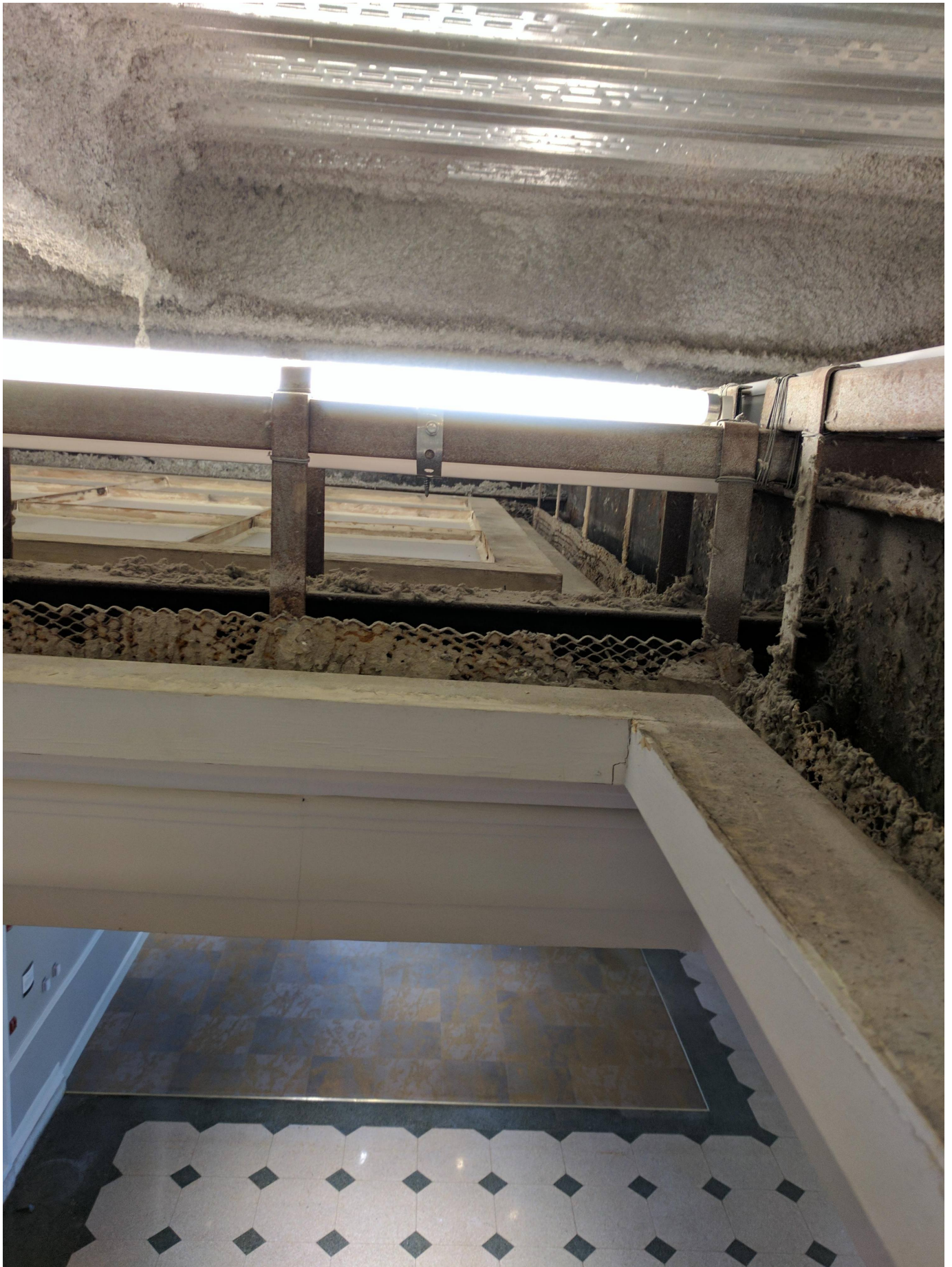
View of laylight attachment method - wood frame relies on plaster and metal lath and metal ties to steel structure for rigidity and stability
