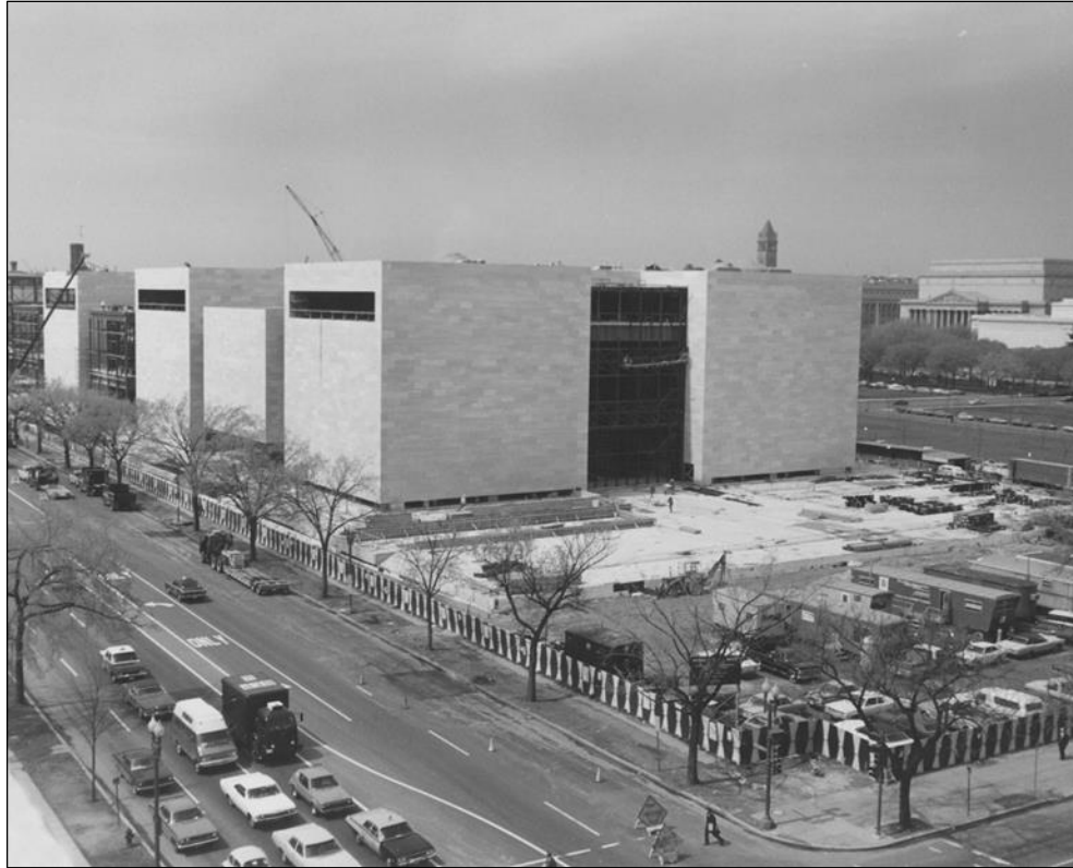
FIGURE 2: NASM AND EAST TERRACE, DURING CONSTRUCTION (1974)
