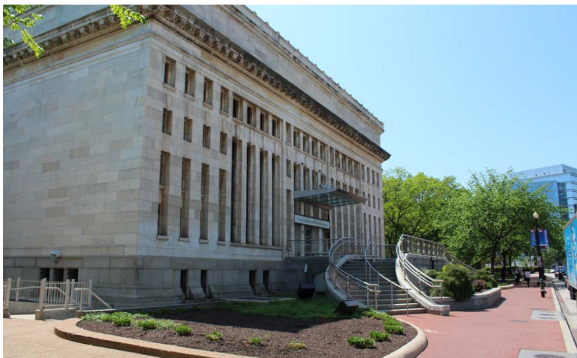
Figure 4: North elevation (including non-original stair and awning), facing southwest
